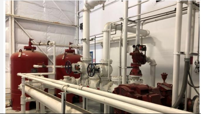
500-gal Ansul tanks connected to the deluge system (top) and hangar drain leading to the underground storage tanks (bottom).
