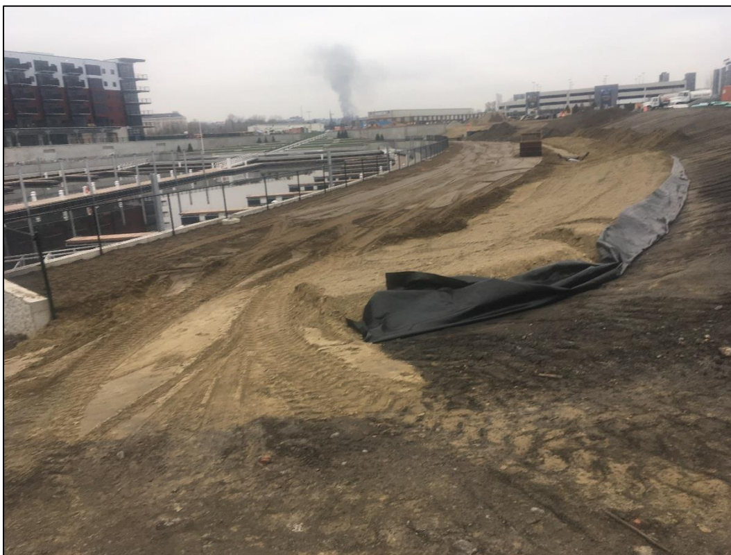
Photo 2. Parcel A – remaining portion being capped, November 2017.
