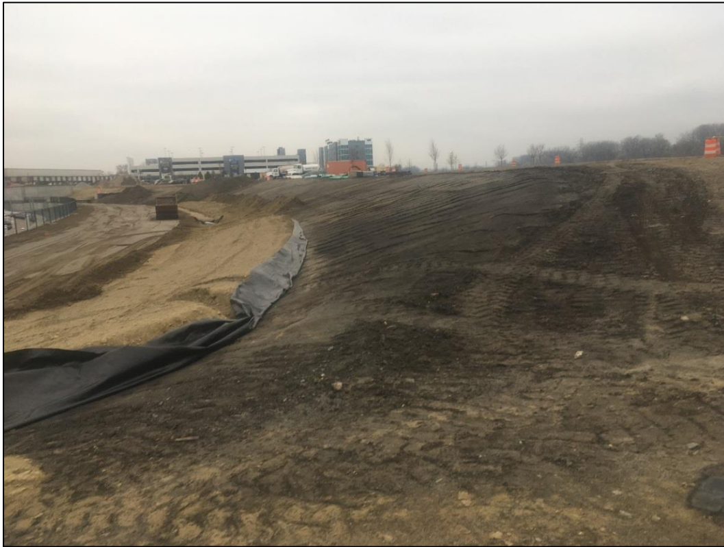
Photo 3. Parcel A – remaining portion being capped, November 2017.
