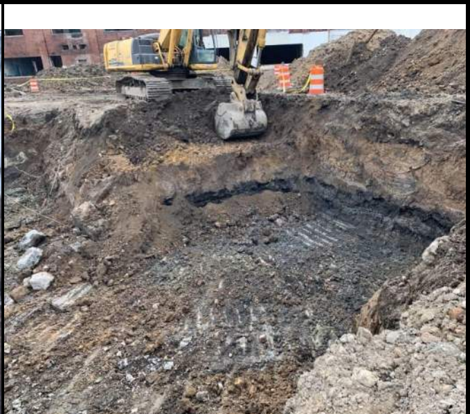
Photograph 2. Excavation of contaminated to on the Syracuse Stamp Property.
