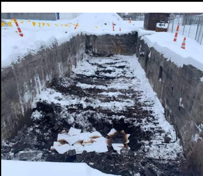
Photograph 1. Basement excavation after the tanks were removed and PEC was attempting to clean out debris to the concrete slab. Broke through and found contamination beneath the concrete slab.
