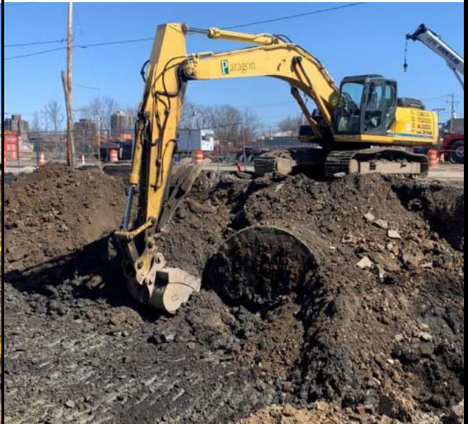
Photograph 4. Uncovering the 10-000 gallon fuel oil UST identified during the spill cleanup work.
