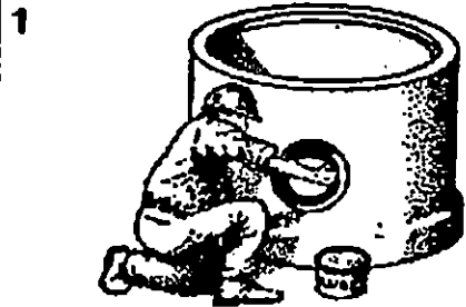
1 CLEAN & LUBRICATE GASKET
