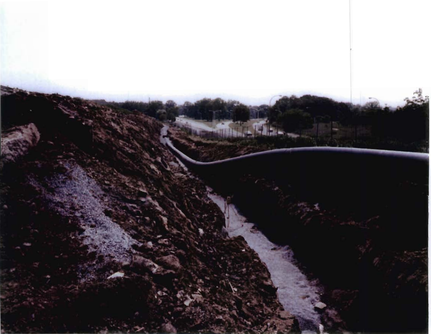
Photo No. 9. Installation of 30" Diameter HDPE Pipe Connection between Ponds B and C. (June 7, 1995)
