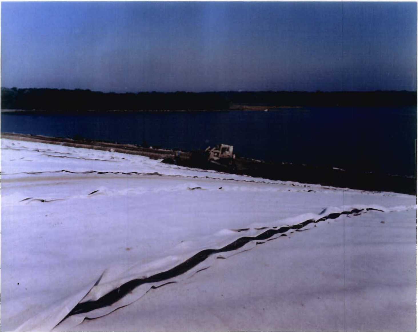
Photo No. 11. Installation of Barrier Protection Material over Geocomposite Layer. (September 27, 1995)
