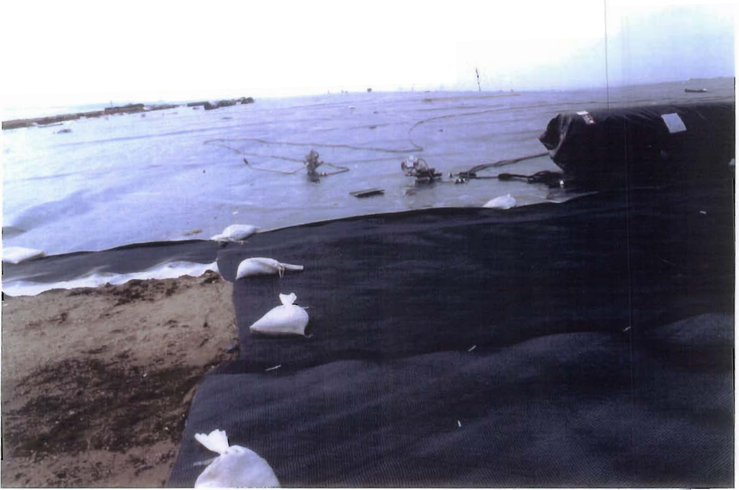
Photo No. 3. Installation of Smooth HDPE Geomembrane at Top of Landfill (November 1, 1995)
