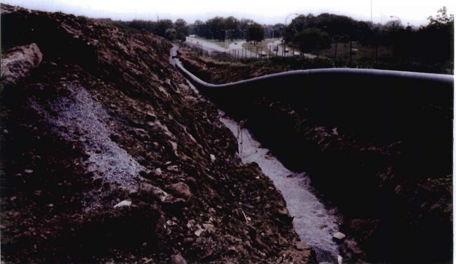
Photo No. 9. Installation of 30" Diameter HDPE Pipe Connection between Ponds B and C. (June 7, 1995)
