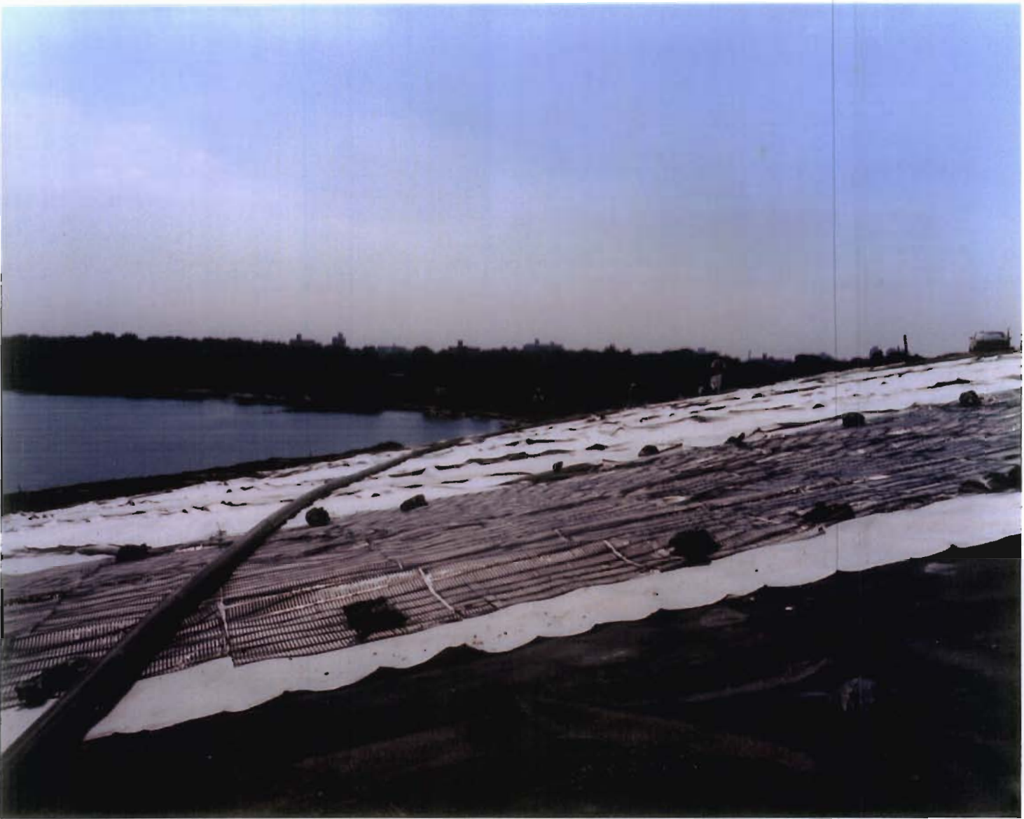
Photo No. 8. LFG Collection Pipe Installation over Geocomposite Layer (with Geogrid Reinforcement). (August 1, 1995)
