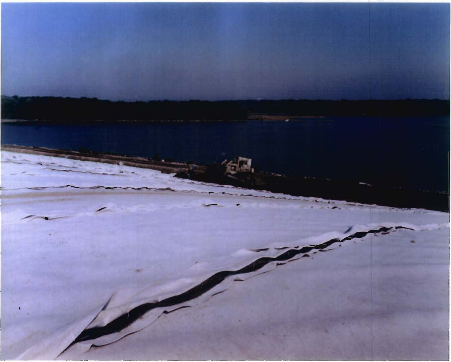
Photo No. 11. Installation of Barrier Protection Material over Geocomposite Layer. (September 27, 1995)
