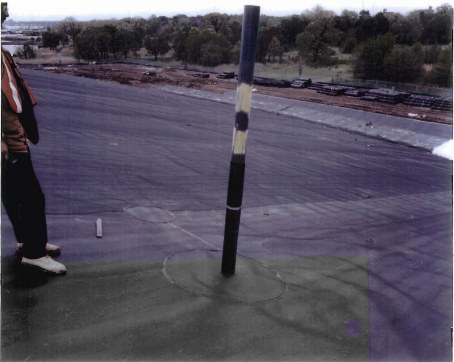
Photo No. 5. Detail of LFG Vent Boot. (May 11, 1995)
