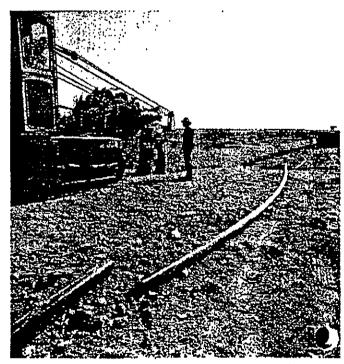
Where the terrain or topography may dictate, Driscopipe 6400 has been joined in a more practical area, then pulled or pushed into place. This has been done with lengths of 1000 feet or more.
