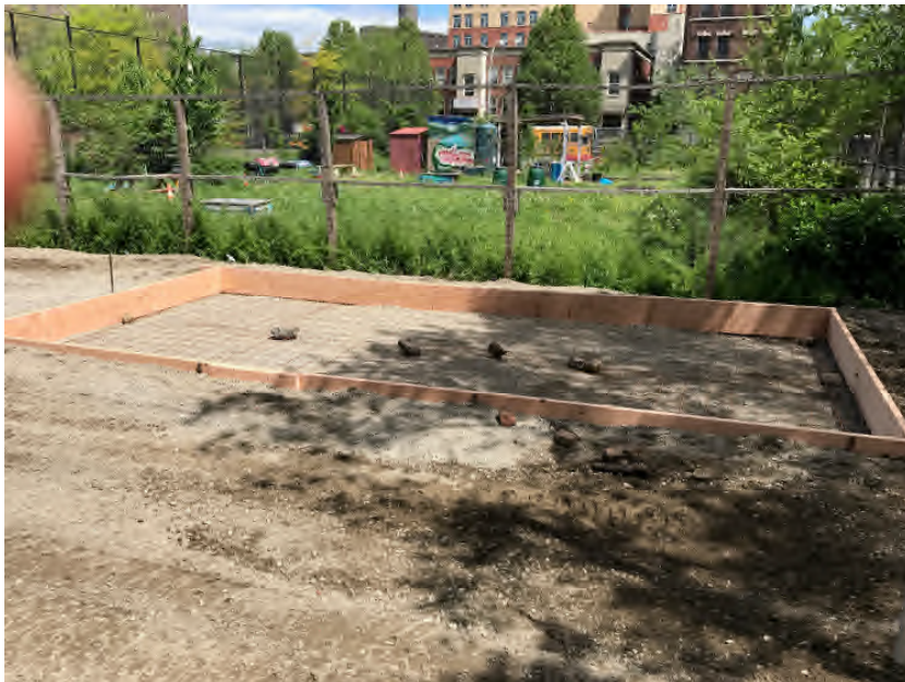
Photograph 24: Construction of 10 x 20 concrete pad at 753 Melrose Avenue.
