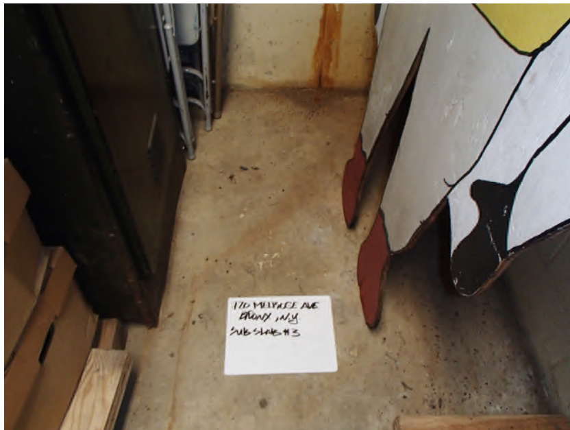
Photograph 8: Sub-slab #3 installation location (720 Melrose Avenue).
