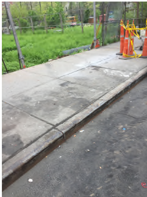
Photograph 16: Fence removal and re-installation at 753 Melrose Avenue.
