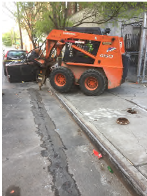
Photograph 18: Curb-cut preparation and installation at 753 Melrose Avenue.
