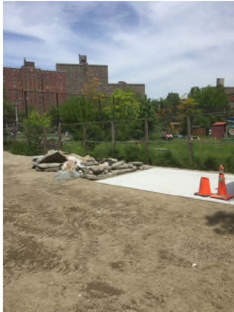
Photograph 25: Concrete pad completion at 753 Melrose Avenue.
