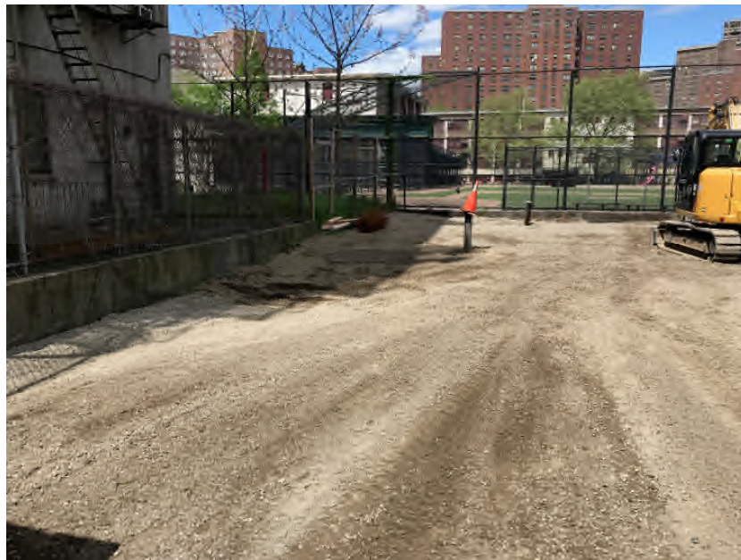
Photograph 26: Completed site grading.
