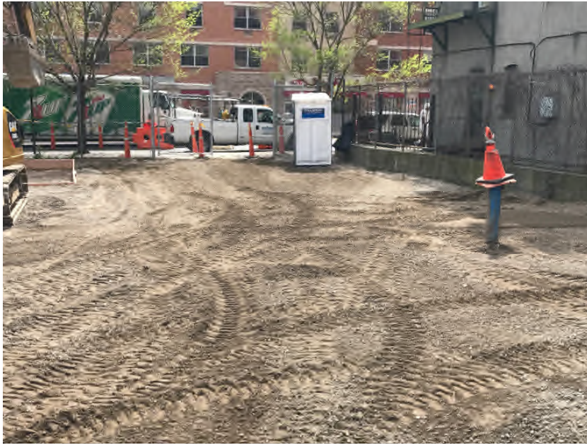
Photograph 23: Site grading at 753 Melrose Avenue.
