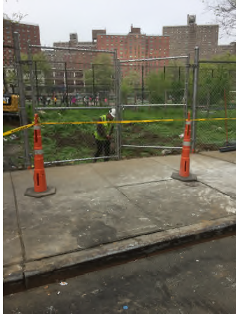
Photograph 17: Fence removal and re-installation at 753 Melrose Avenue.
