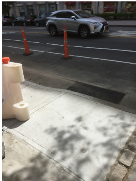
Photograph 20: Sidewalk flag replacement at 753 Melrose Avenue.
