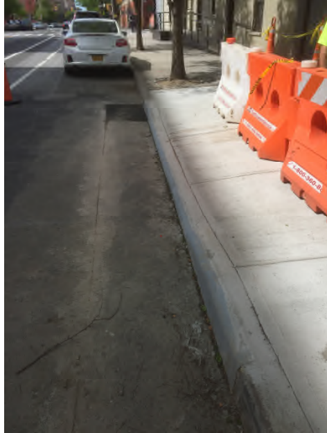
Photograph 19: Completion of sidewalk curb-cut at 753 Melrose Avenue.
