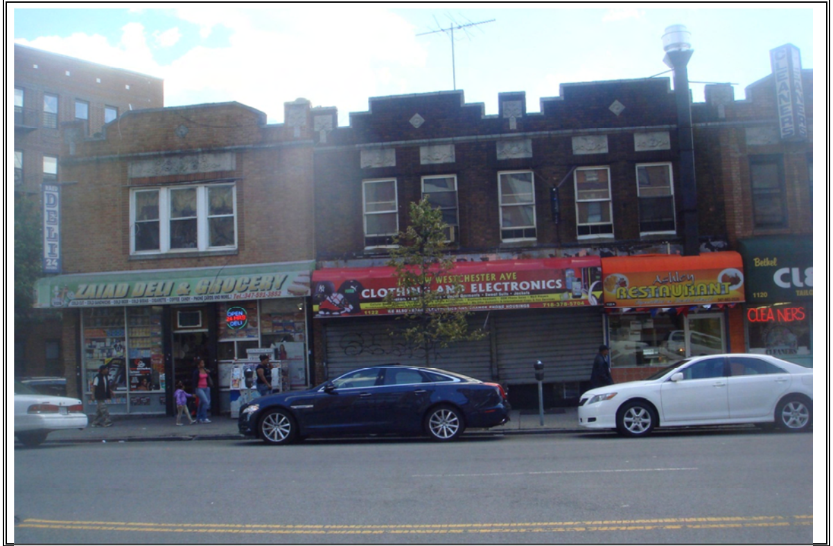
Photograph Number 5: Property located to the east – Residential/Stores
