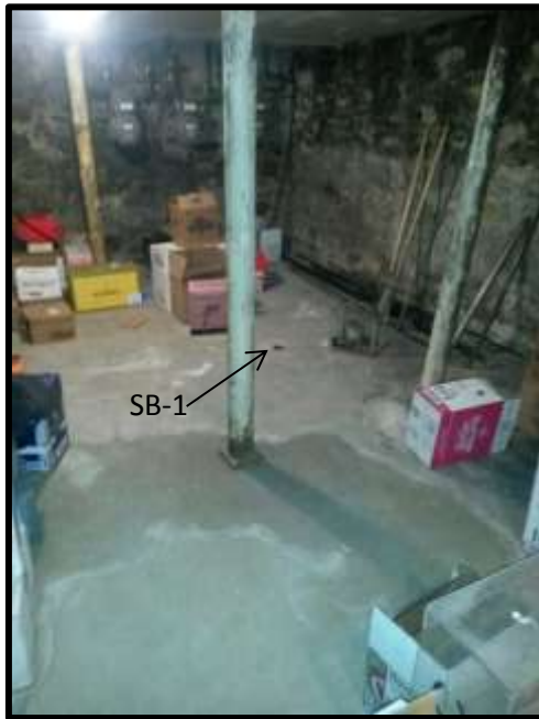
2. View depicting the location of boring SB-1.
