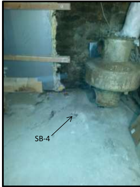
5. View of the location of boring SB-4.
