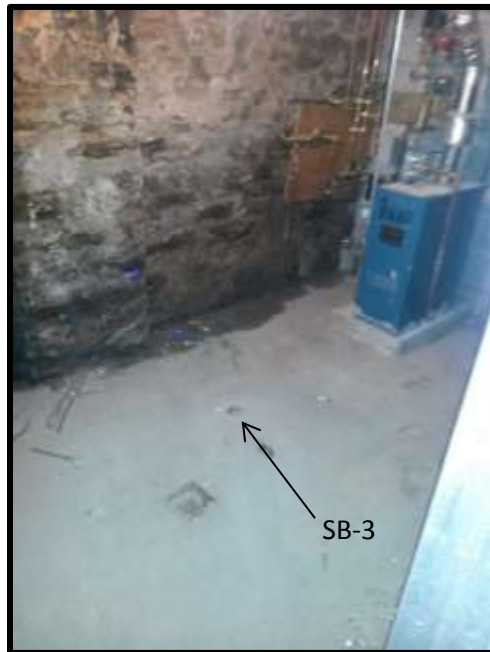
4. View depicting the location of boring SB-3.
