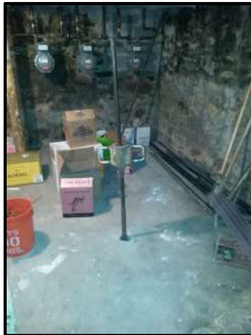
6. View of the hand boring equipment.
