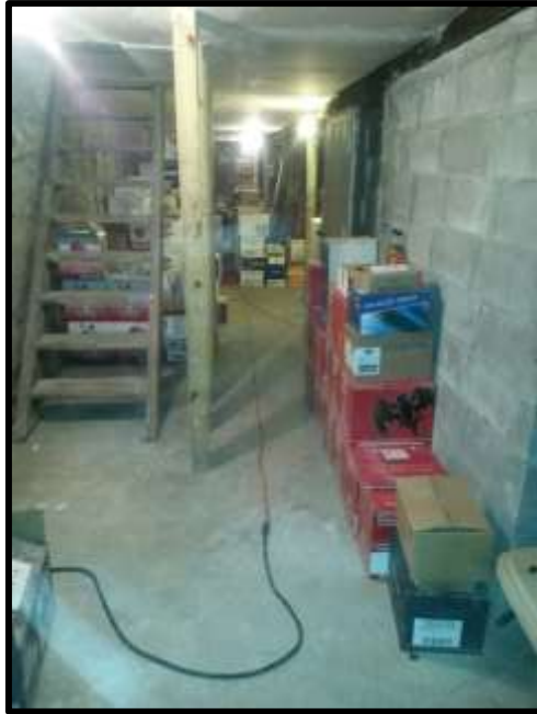
1. View of the basement area in the subject building.
