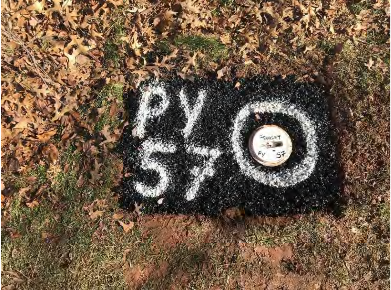
Typical Top of PVC Guide Pipe/Collar
