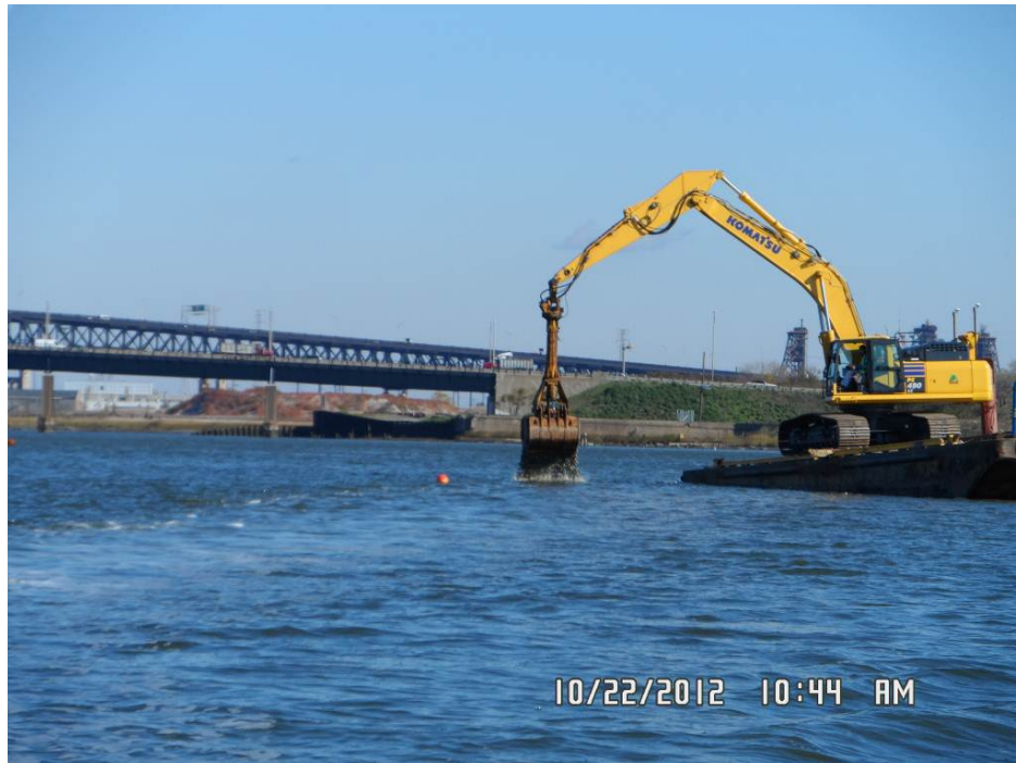
Photo 1: Mechanical placement of armor in Cap Area 17.
