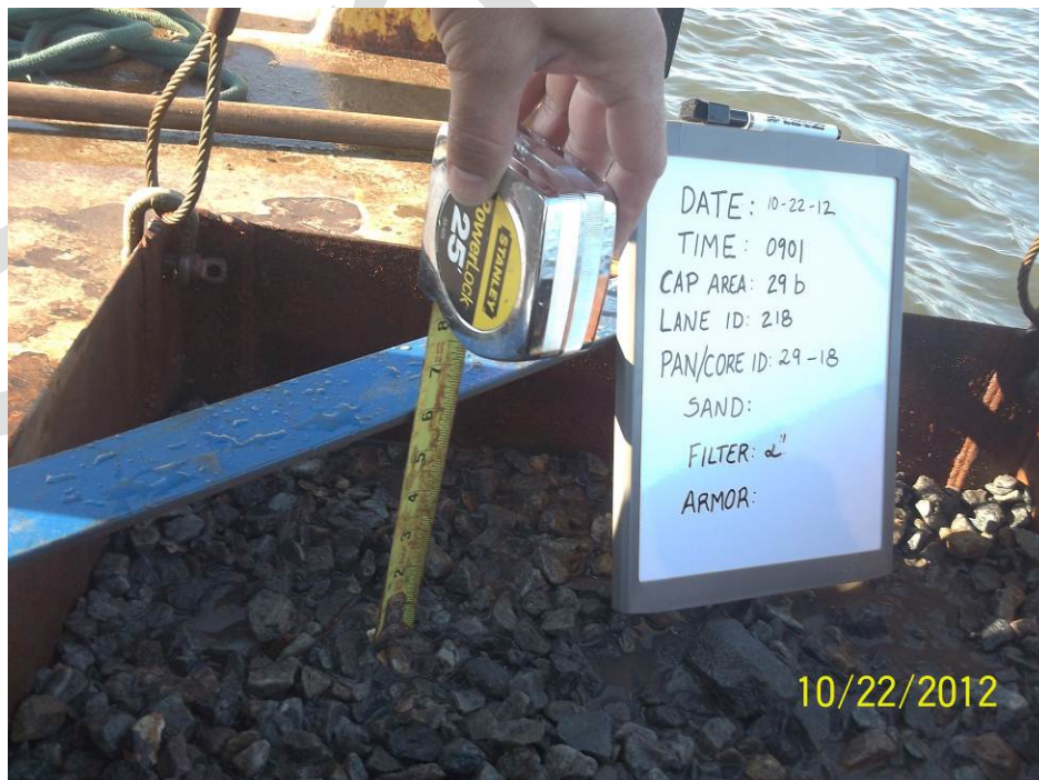
Photo 2: Filter thickness verification in Cap Area 29B.
