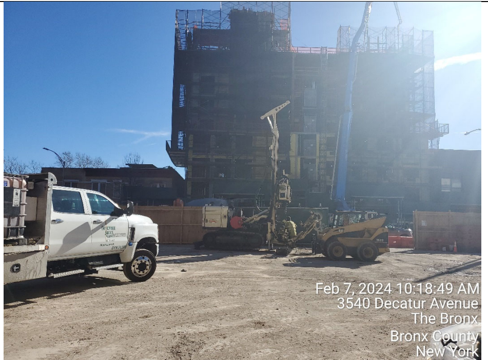
Photo 3: View of bedrock well installation at MW-11
