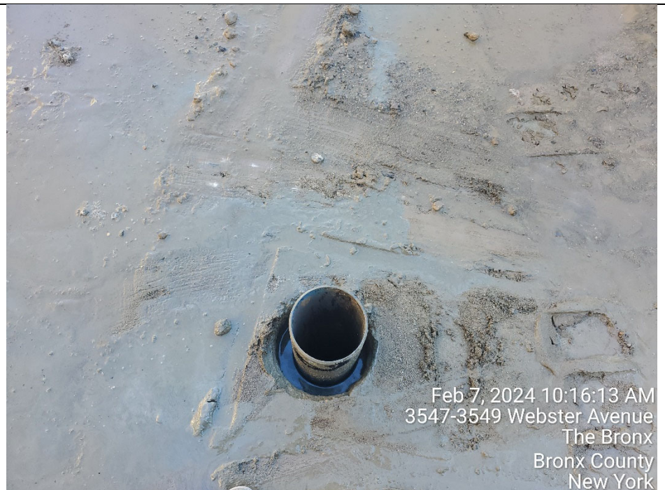
Photo 2: View of bedrock well installation at MW-13
