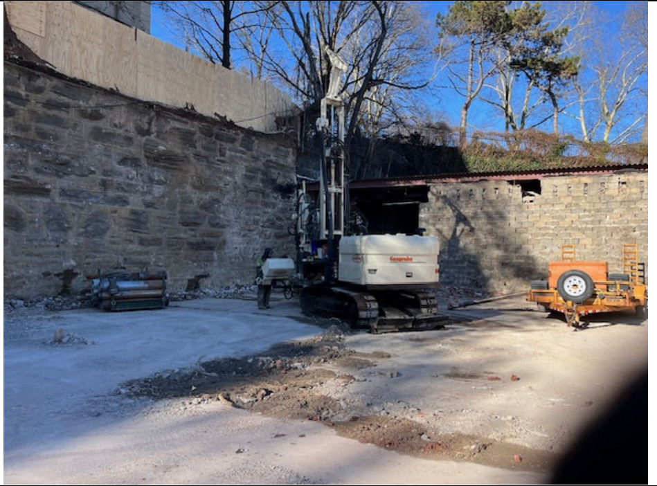
Photo 2: View of bedrock well installation at MW-9
