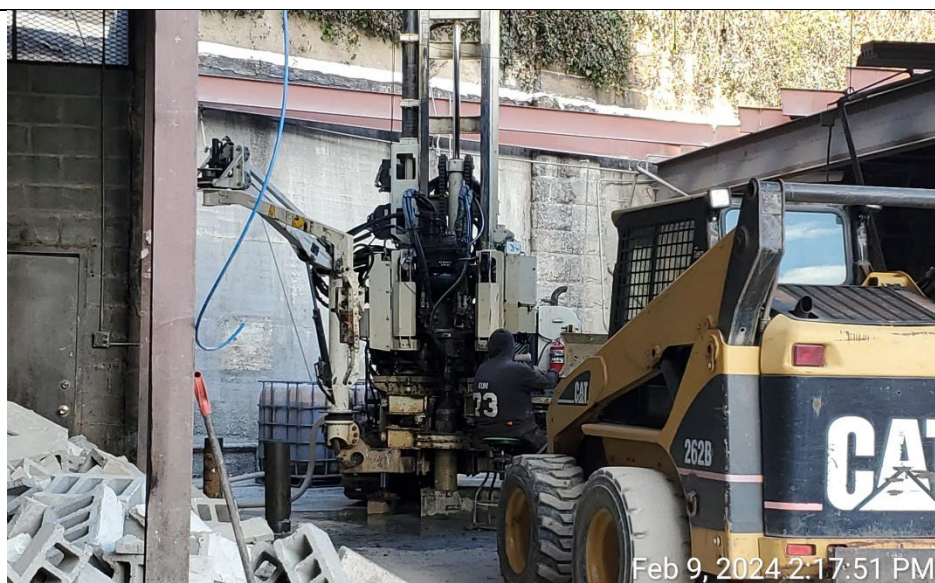
Photo 4: View of bedrock well installation at MW-6.
