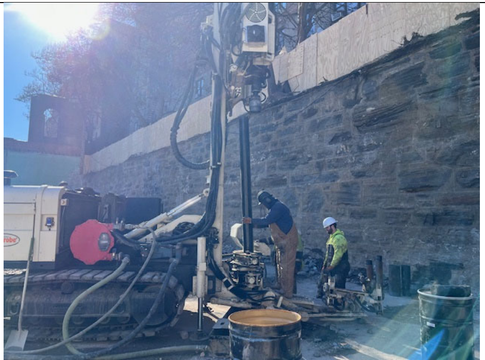
Photo 3: View of bedrock well installation at MW-9
