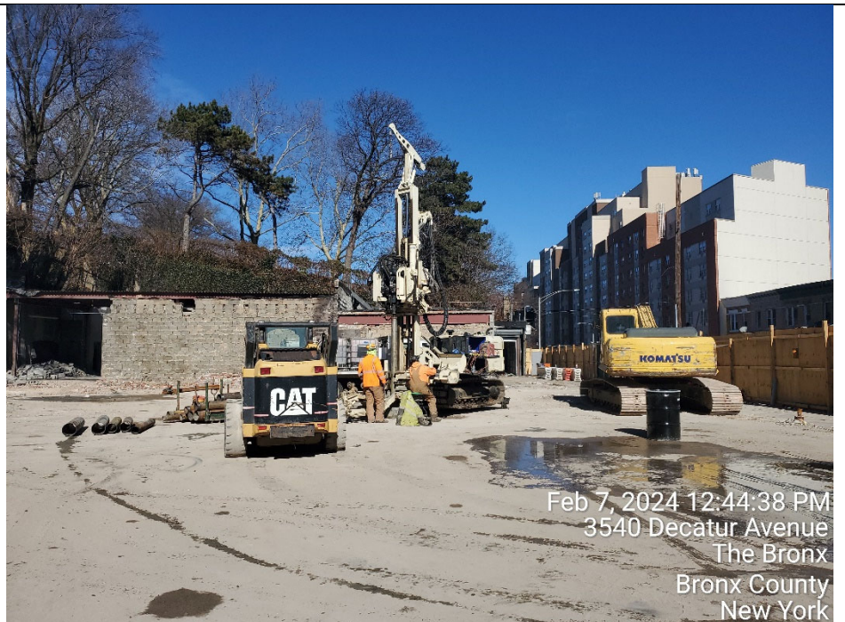
Photo 4: View of bedrock well installation MW- 10
