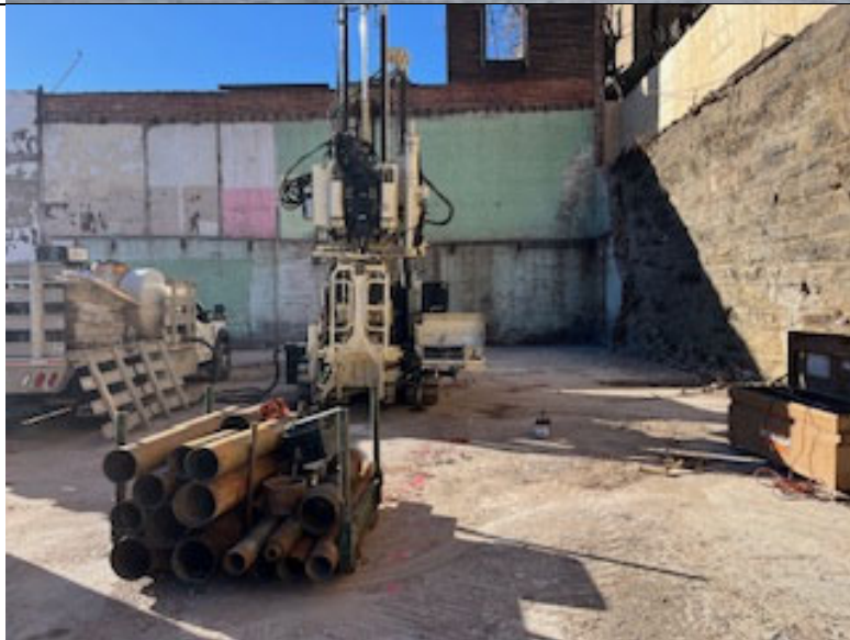
Photo 3: View of bedrock well installation at MW-12
