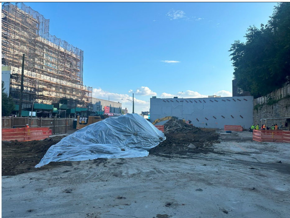
Photo 5: View of site at the end of the work day with soil stockpile covered with plastic sheeting, facing south.
