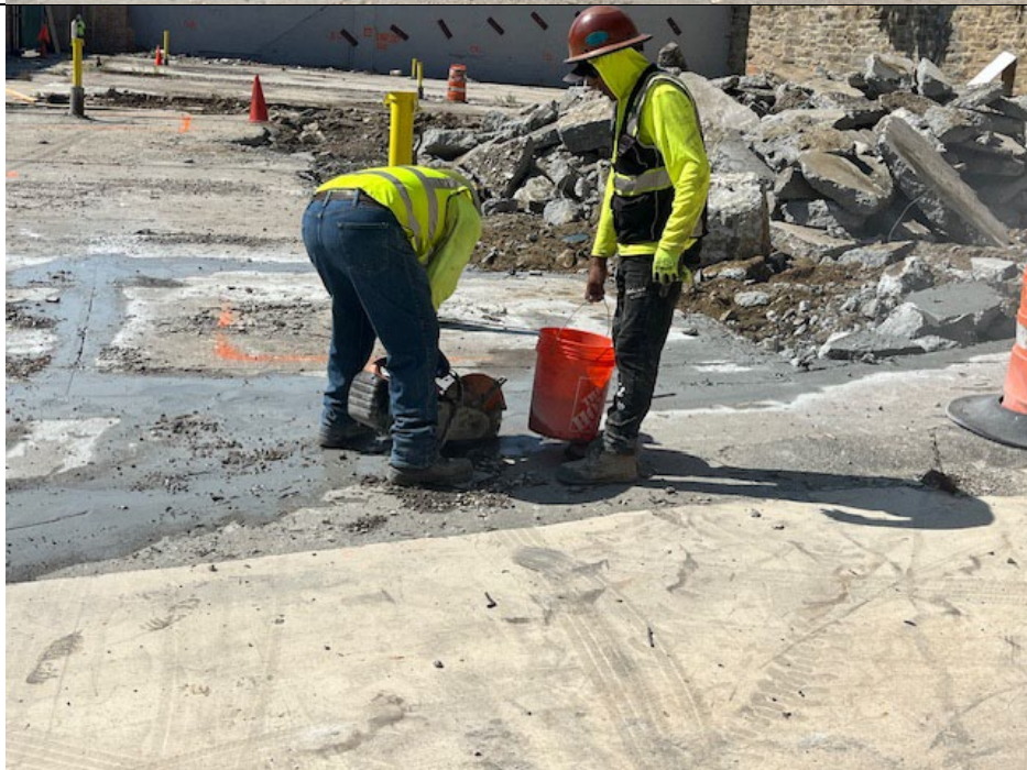
Photo 4: View of saw cutting and wetting down concrete
