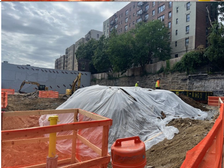
Photo 6: View of stockpile covered in plastic sheeting and monitoring wells protected with barriers
