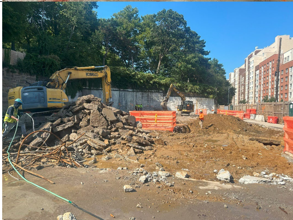
Photo 4: View of concrete slab breaking in Grid A and soil stockpiling in Grid B. Workers use hoses with fresh water to suppress dust from both work activities.
