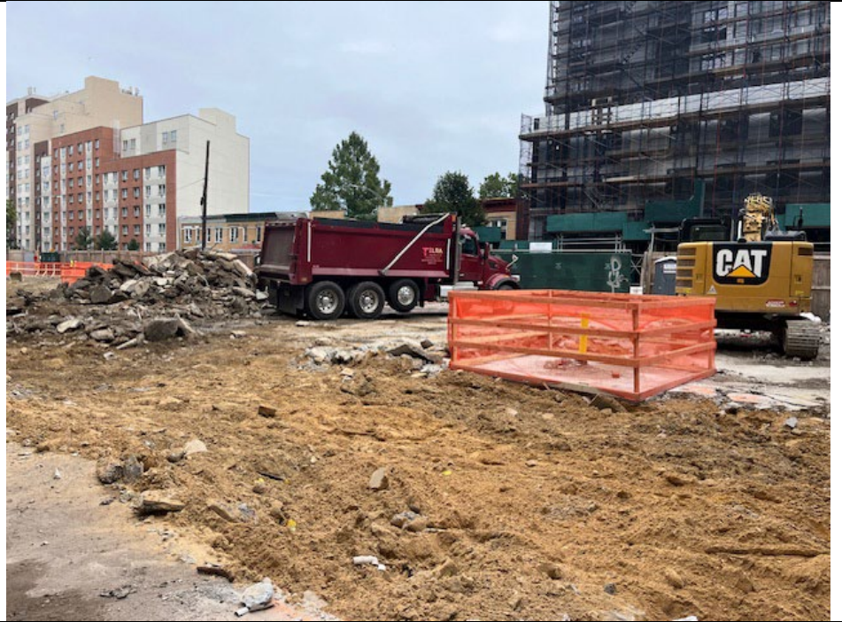
Photo 2: View of loading out concrete for export to Mount Materials, looking northeast.
