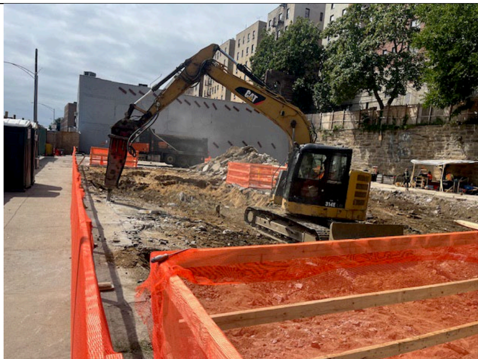
Photo 3: View of concrete slab breaking in Grid A and soil stockpiling in Grid B.
