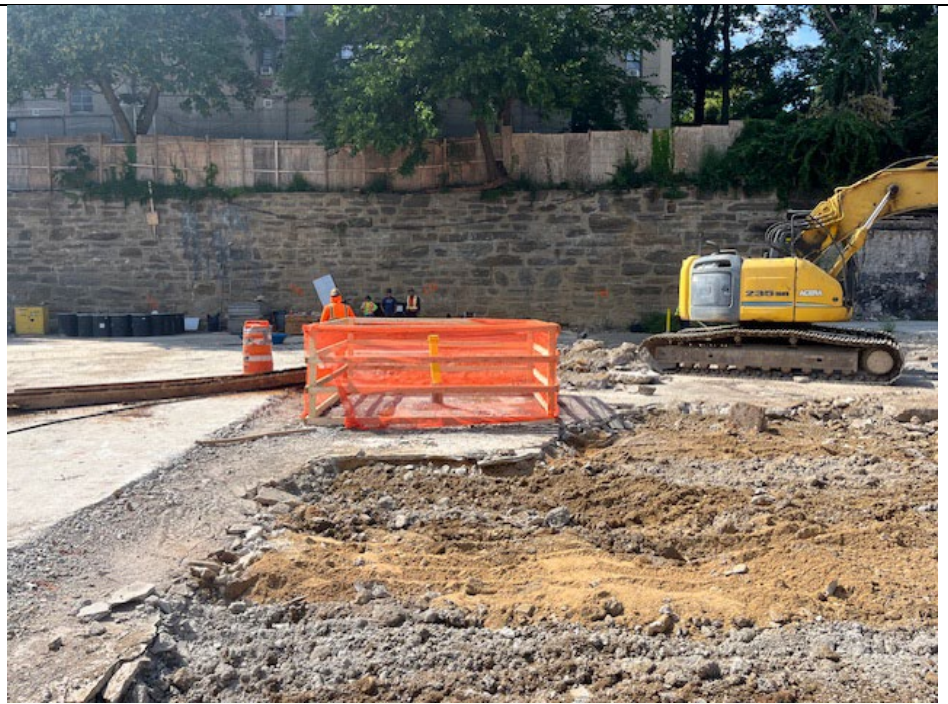
Photo 5: View of installed protection around monitoring wells
