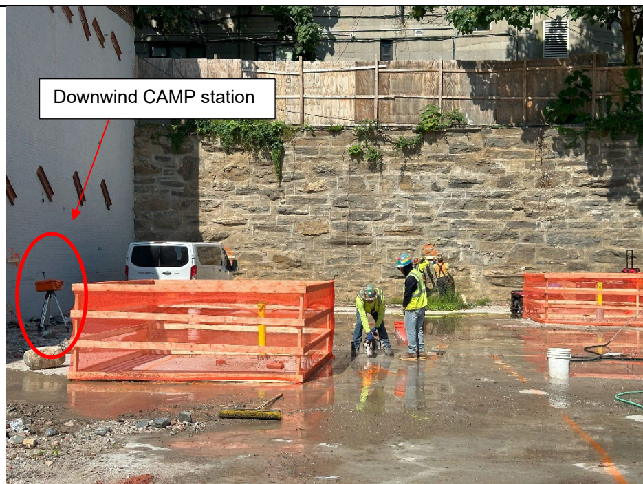
Photo 3: Workers saw cutting the concrete slab using water to suppress dust, downwind CAMP station in view.
