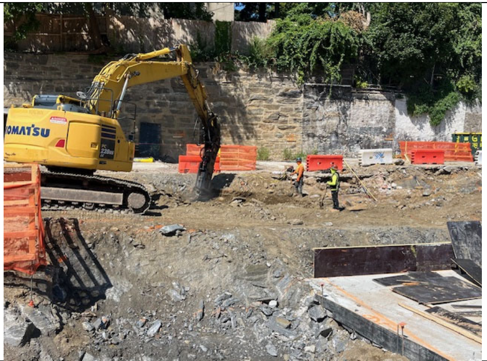
Photo 3: View of breaking bedrock in Grid B.
