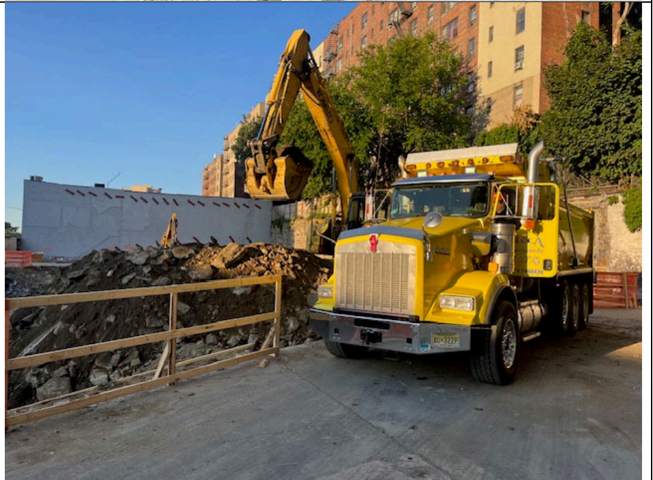
Photo 2: View of soil being loaded for export to Baysshore Soil Management.
