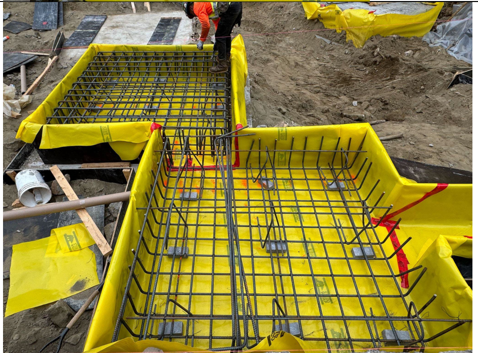
Photo 6: Installation of vapor barrier and rebar by EP-15
