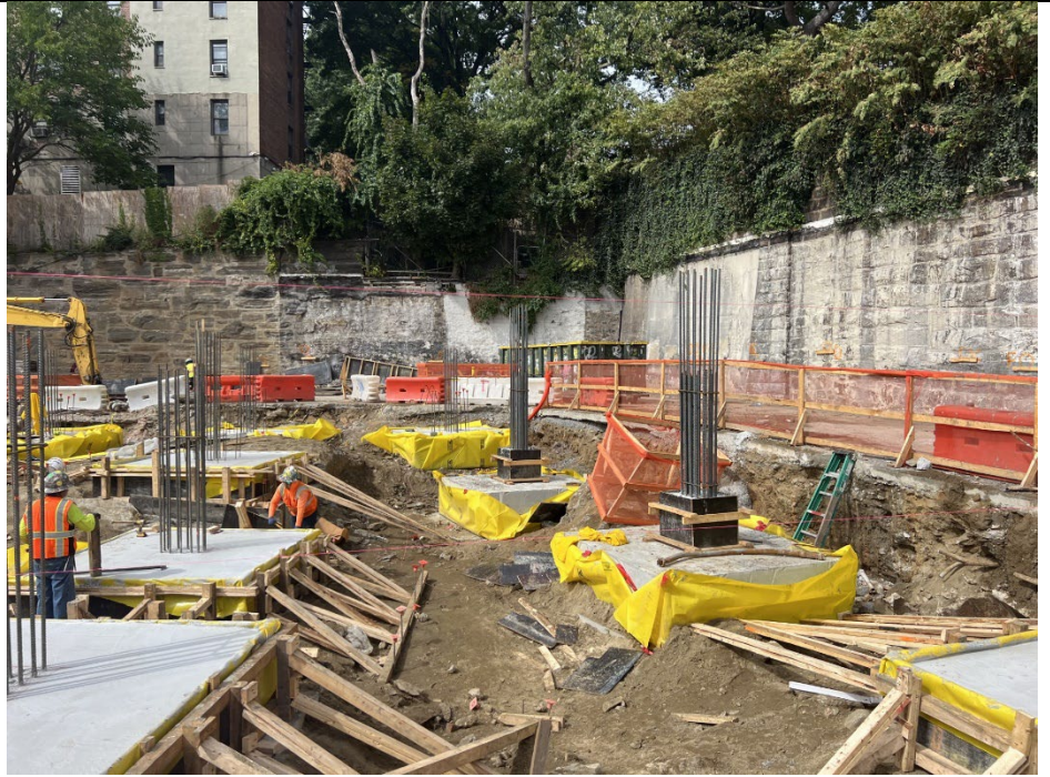
Photo 3: Rebar and vapor barrier installation at footings, westward view
