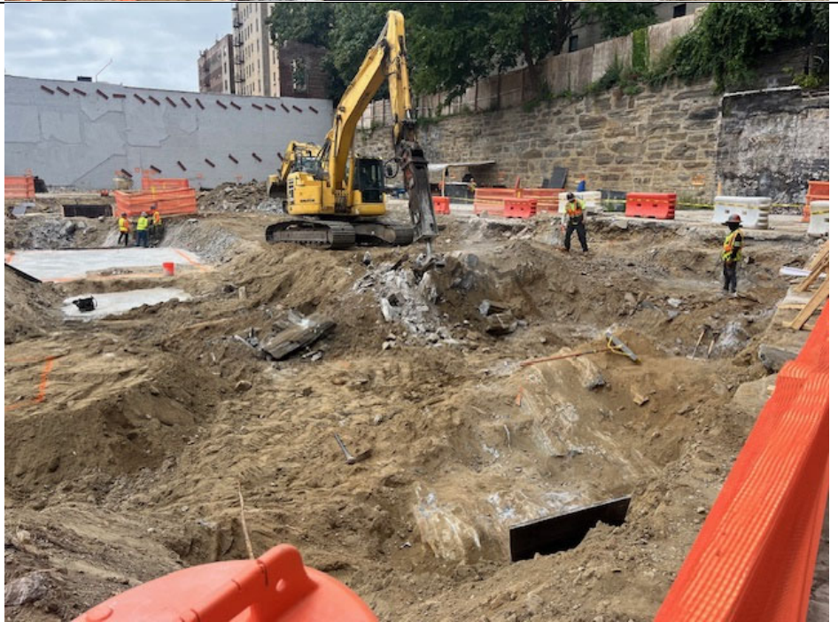
Photo 4: View of bedrock breaking in central portion of site
