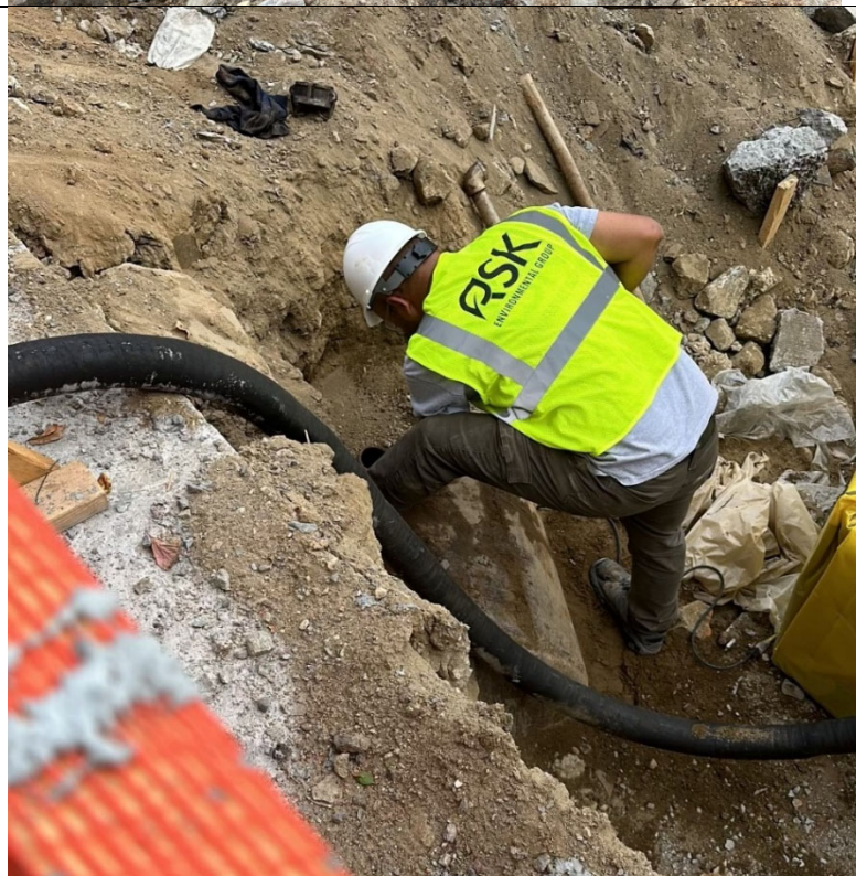
Photo 6: Liquid contents being removed from 550-gallon UST
