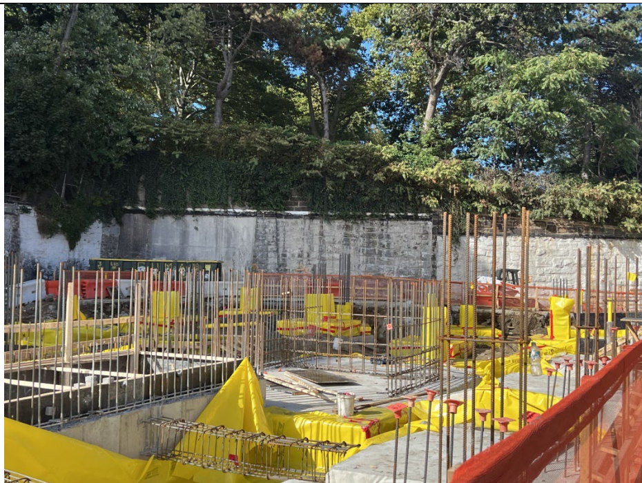
Photo 3: Rebar and vapor barrier installation at footings, view facing north
