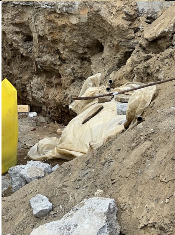
Photo 8: UST covered in plastic sheeting at the end of the workday.
