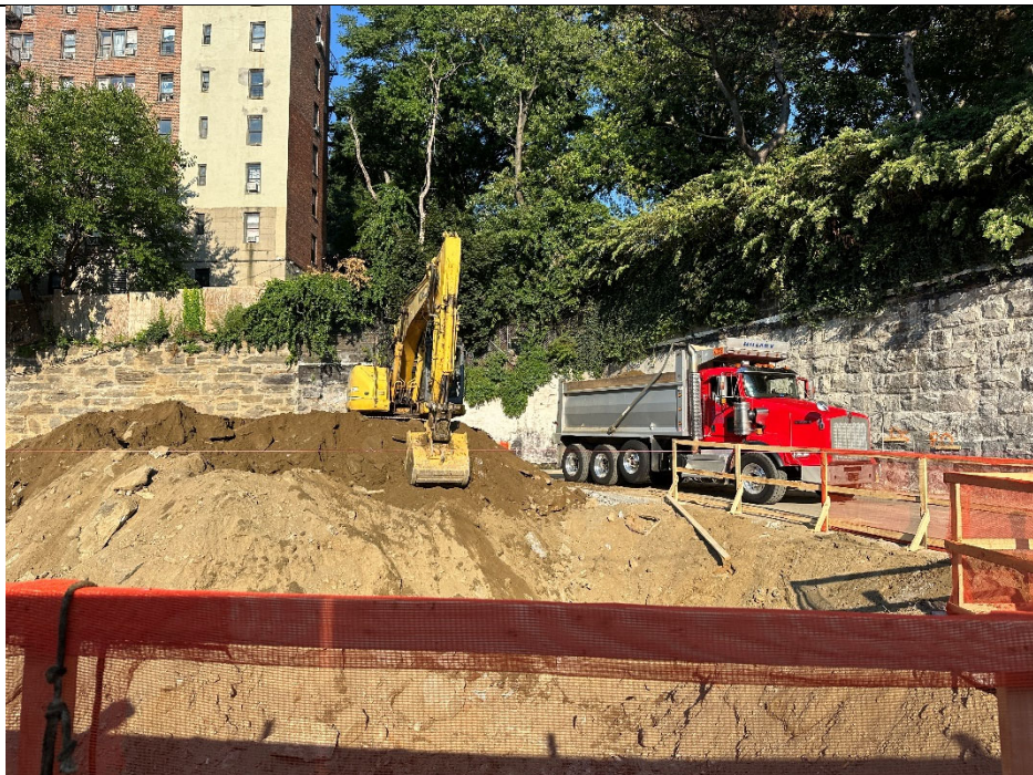
Photo 3: View of soil being loaded for export to Bayshore Soil Management.
