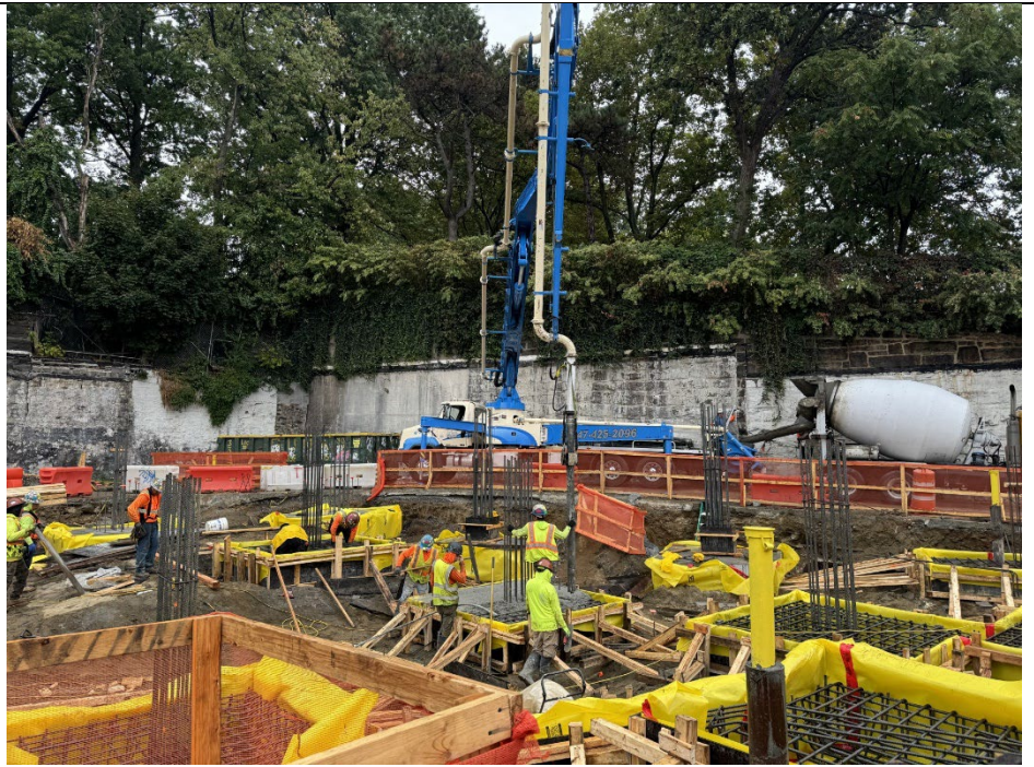
Photo 3: Elevator pit filled with concrete and covered with vapor barrier.
