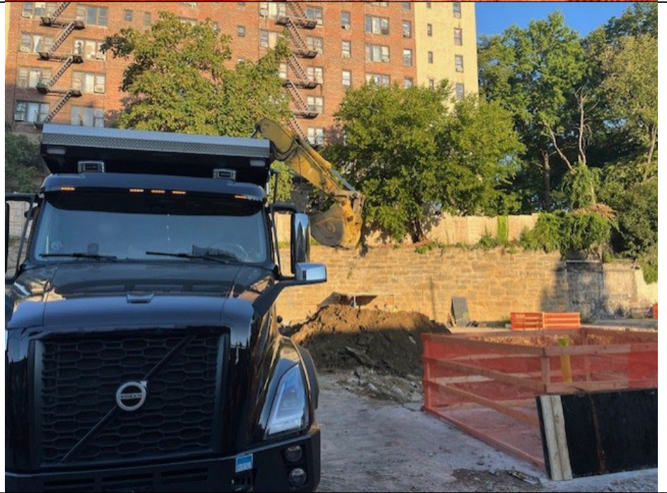
Photo 2: View of soil being loaded for export to Bayshore Soil Management.
