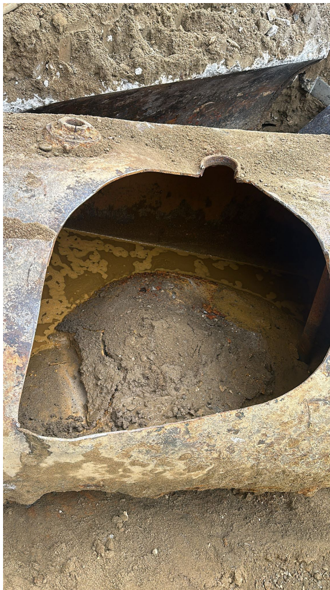
Photo 2: Contents of the underground oil tank excavated by RSK Environmental
