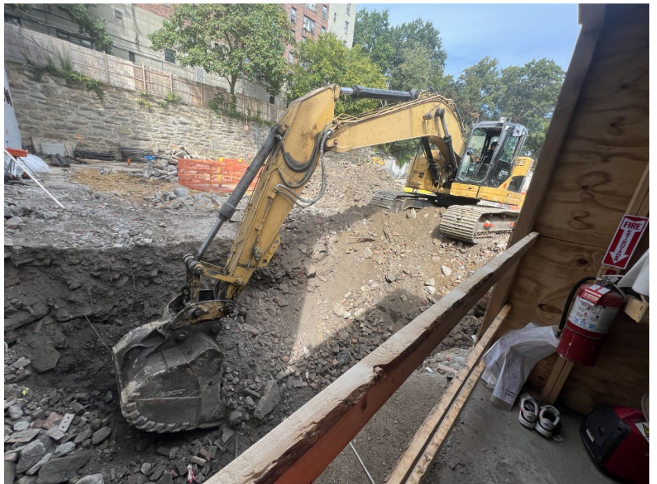
Photo 2: Excavation in preparation for footing installment at Grid A
