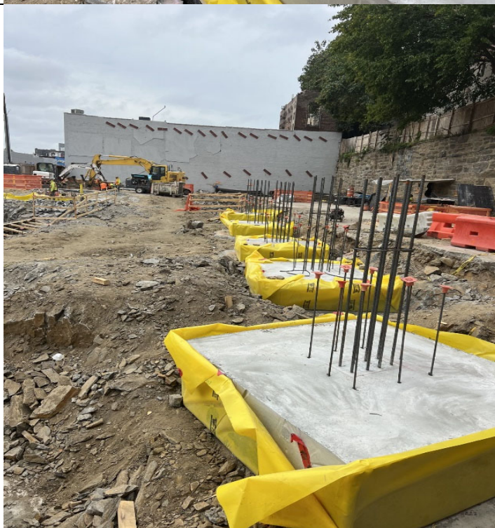
Photo 4: Southward view of site showing rebar formwork
