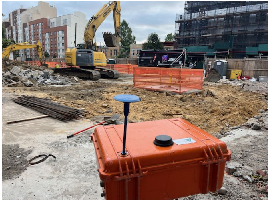
Photo 2: View of downwind CAMP station and soil being loaded for export to Bayshore Soil Management.
