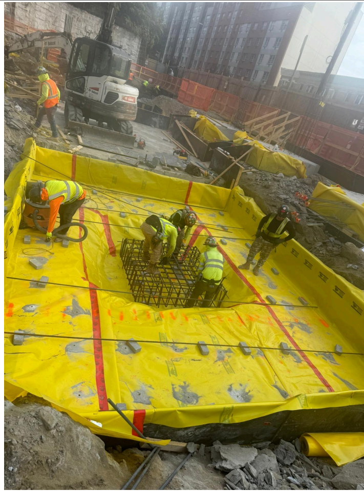
Photo 3: After laying down the vapor barrier in the elevator pit)
