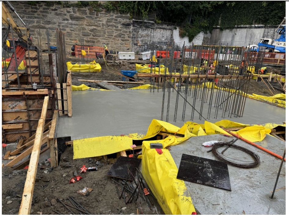
Photo 4: Continued installation of rebar by Raptor Construction in the elevator footing
