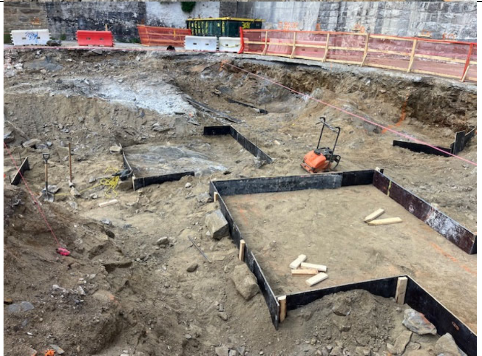
Photo 4: View of installed formwork in Grid B.
