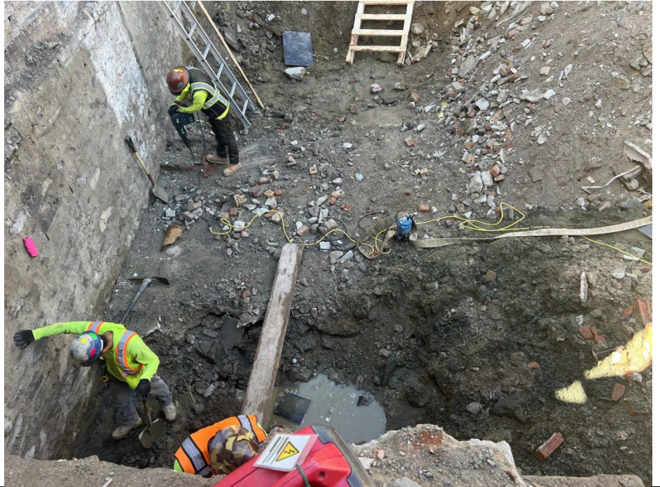
Photo 1: Rain water removal at Grid A, southeastern most corner of the site
