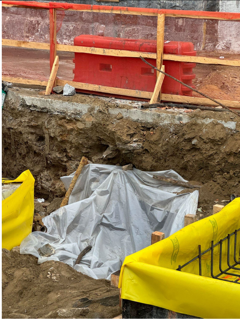
Photo 3: RSK Environmental covers oil storage tank in plastic sheeting
