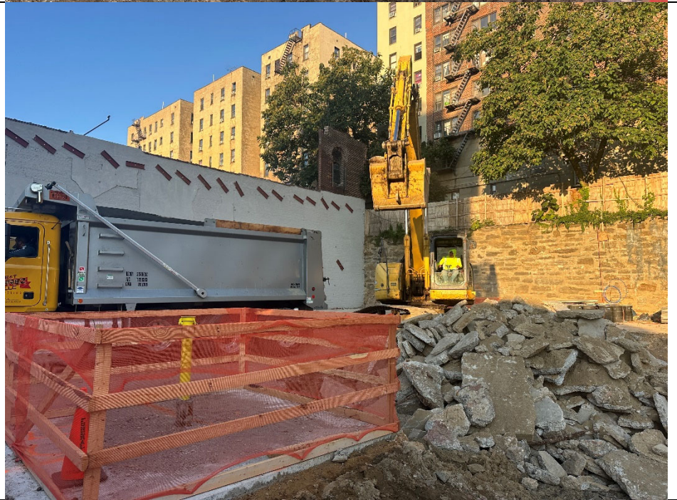
Photo 2: View of C&D being loaded for export to Mount Materials.
