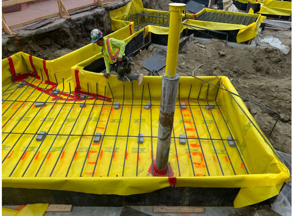
Photo 8: Installation of vapor barrier and rebar by MW-7 (cont'd)
