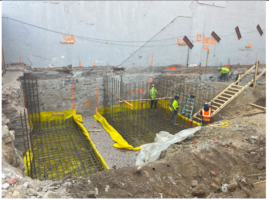
Photo 3: Overview of Grid A footings and rebar installation. Area of anticipated concrete pouring.
