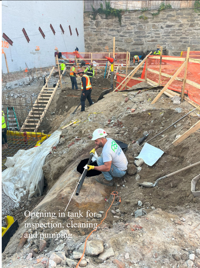
Photo 4: RSK opening and assessing the UST discovered 10/1, determined to be a 14'x5' 3000-gallon tank contained mixed oil. The contents of the tank were pumped halfway and then recovered.
