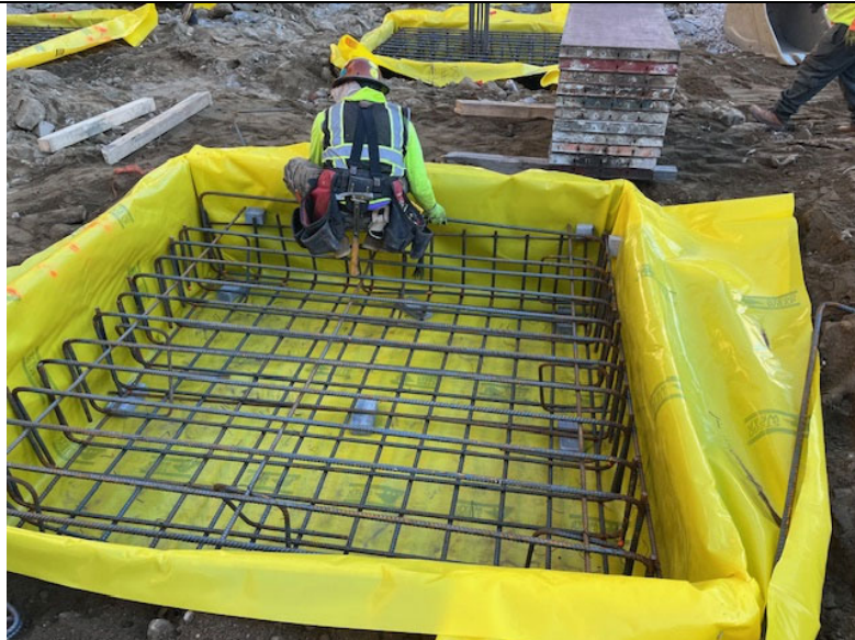
Photo 3: View of installed Stego Wrap-20 mil vapor barrier for footing and rebar installation
