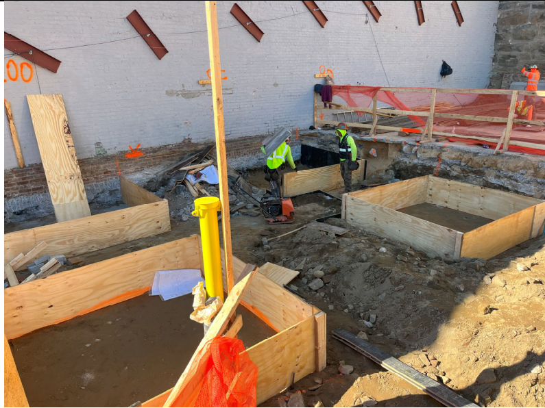
Photo 3: Overview of Grid A footings and rebar installation.
