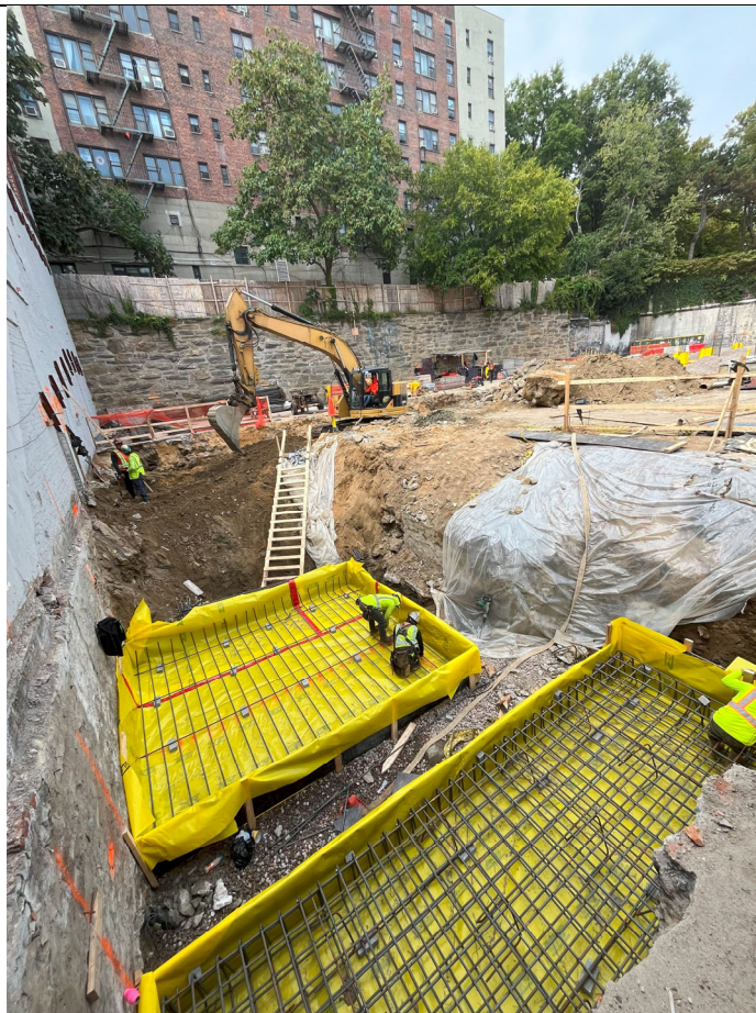
Photo 5: Vapor barrier (Stego Wrap-20 mil) installation and backfilling of RCA in Grid A, facing South at end of workday
