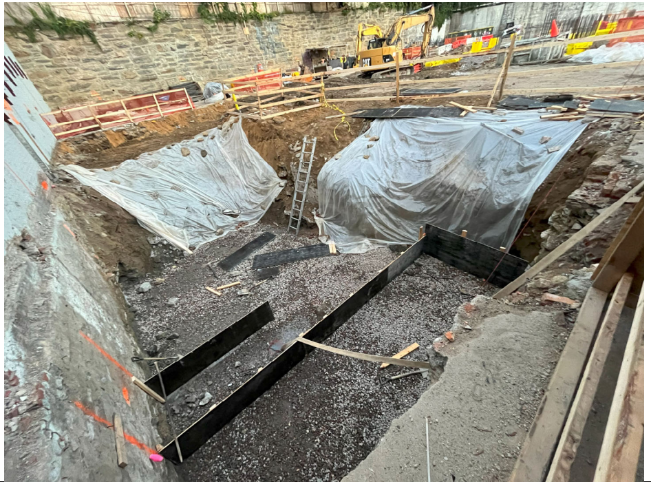
Photo 1: Footings installation in Grid A facing South.
