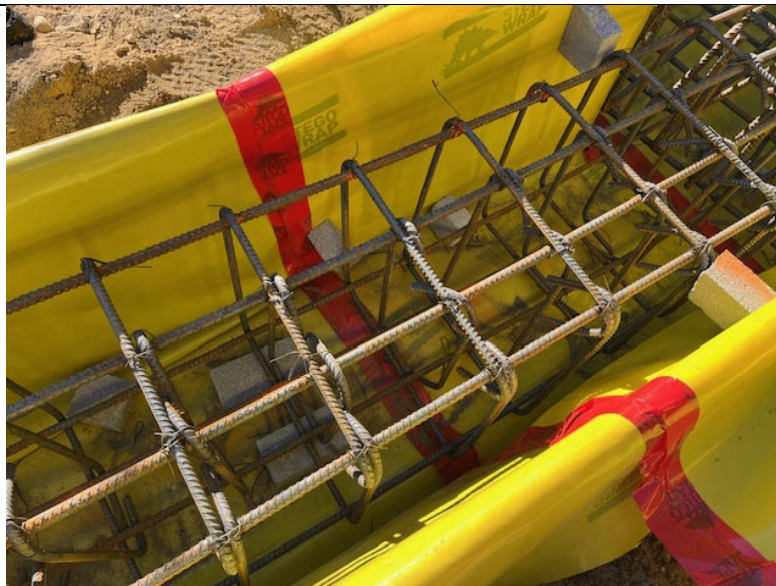
Photo 4: View of installed Stego Wrap-20 mil vapor barrier and Stego tape
