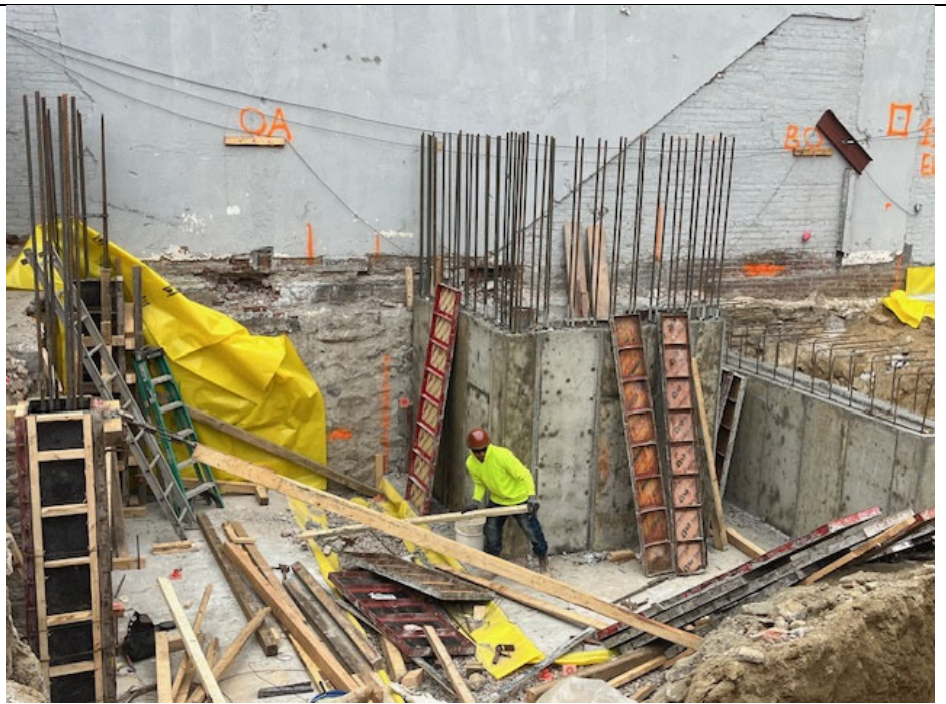
Photo 3: View of Raptor Concrete removing formwork
