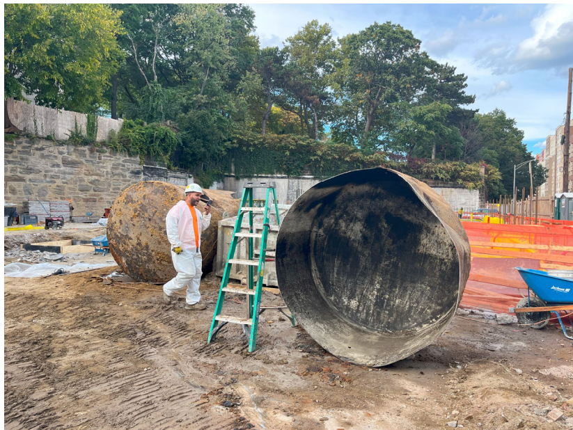
Photo 6: Cross section of emptied UST during removal.
