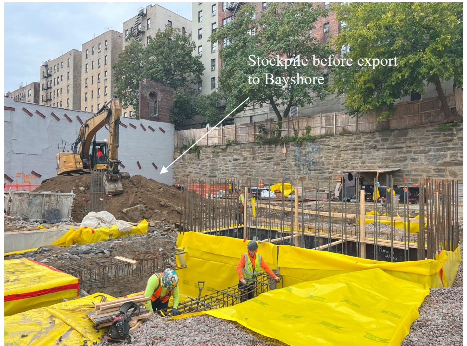
Photo 1: Footings and vapor barrier installation in Grid A facing South.
