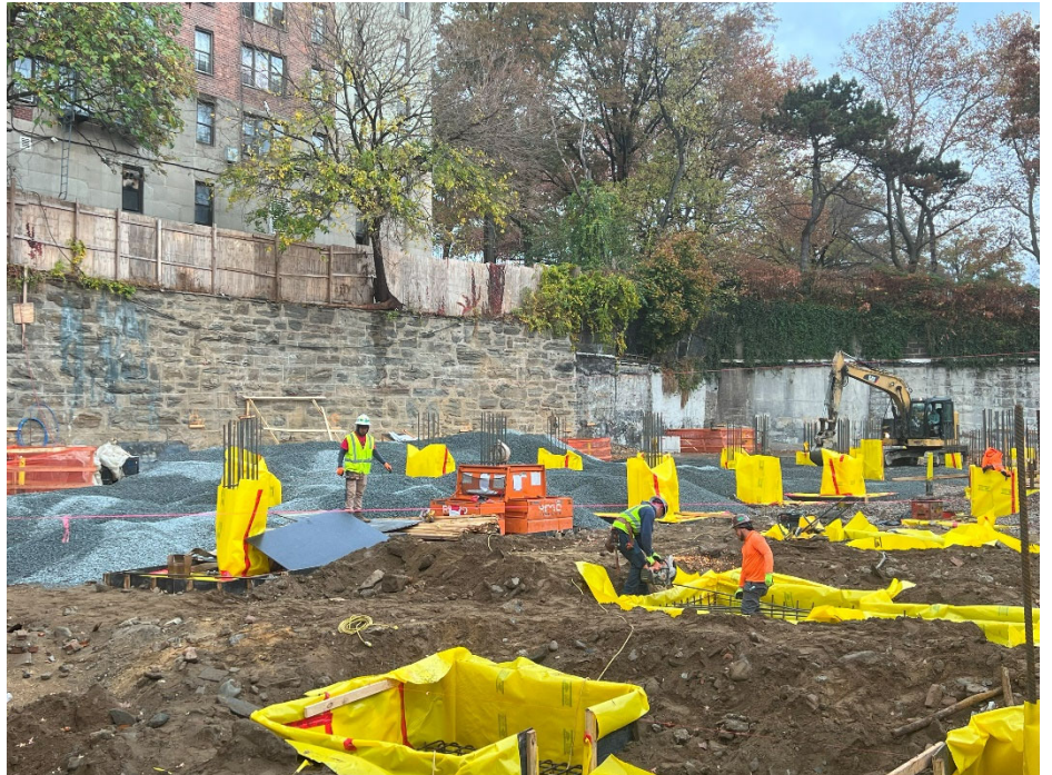
Photo 2: Gravel backfill imported, view facing north.
