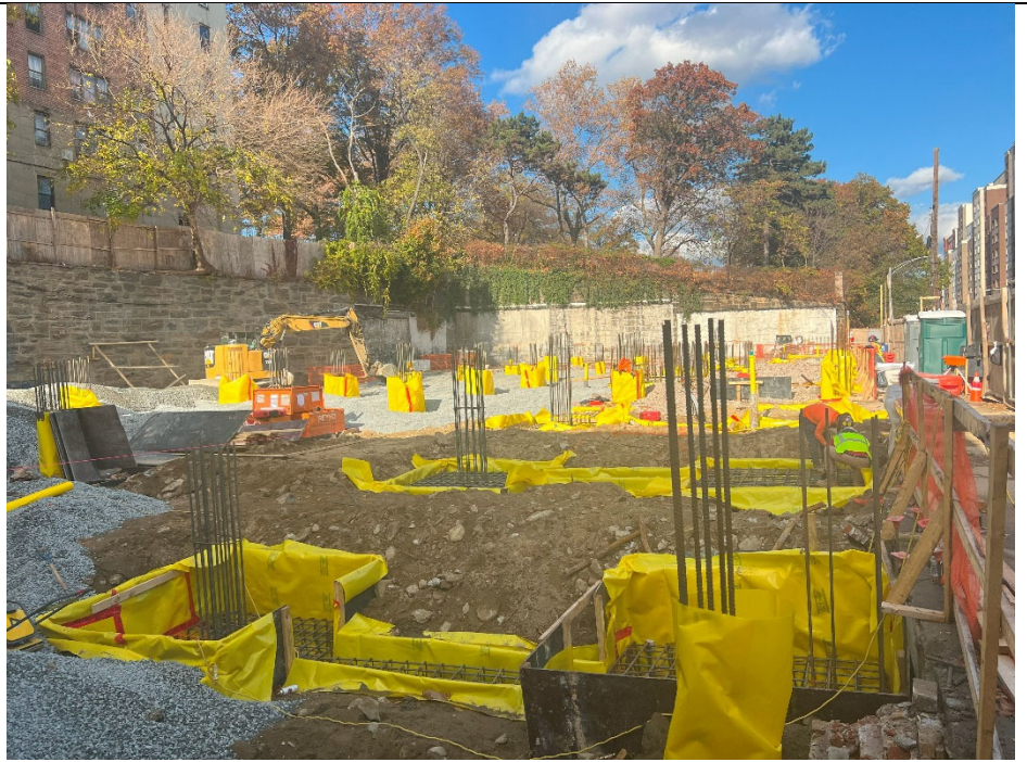
Photo 5: Footing installation, view facing north.
