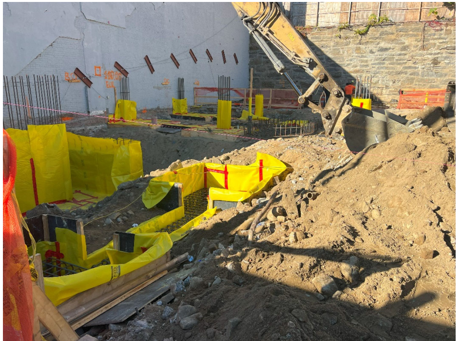
Photo 2: Installation of footing with Stego wrap vapor barrie, view facing southwest.
