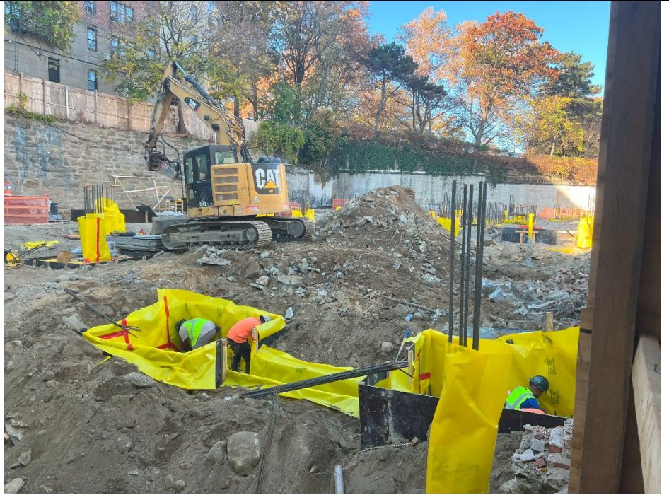
Photo 3: Stego wrap installation of footing to the south of MW-4 in Grid B along Webster Avenue, view facing north.
