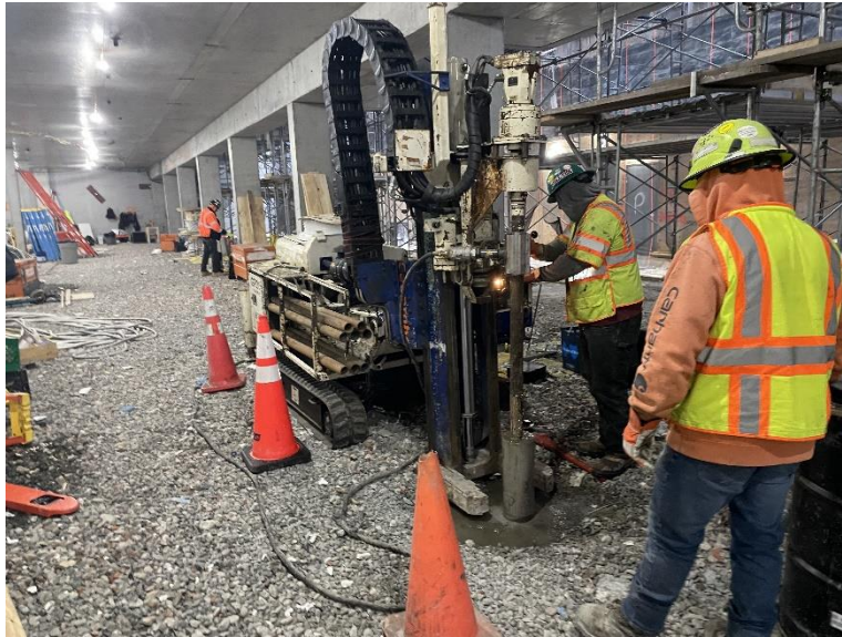
Photo 1: View of ADT drilling MW-15D, facing southwest.
