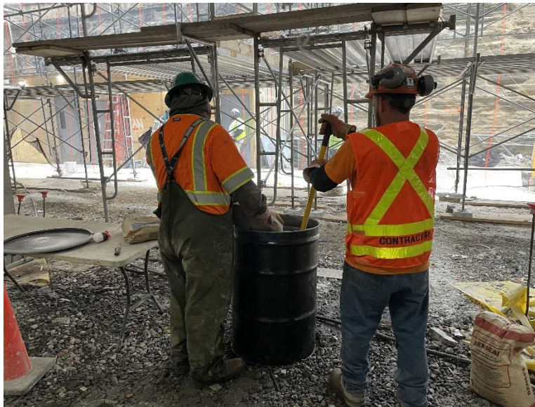
Photo 2: View of ADT grouting the borehole to prepare for MW-15I installation, facing west.
