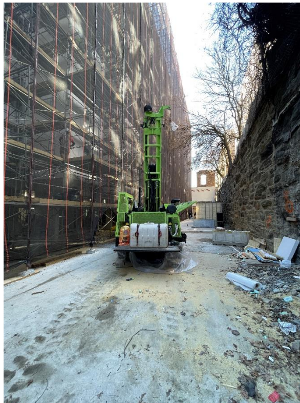
Photo 2: View of ADT set up to install MW-14D, facing south.
