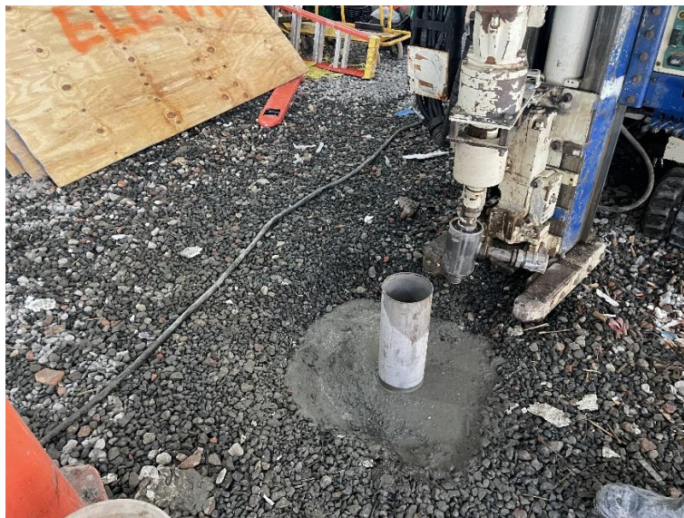
Photo 2: View of the casing set at MW-15D, facing southeast.
