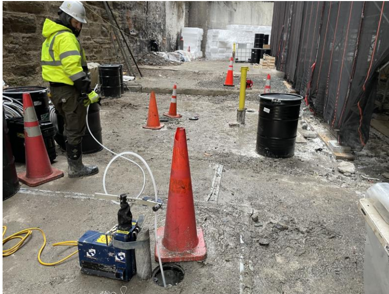
Photo 1: View of Haley & Aldrich developing MW-16D, facing north
