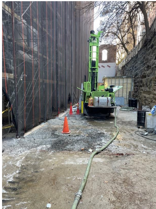
Photo 2: View of sonic drill rig setup on MW-16D, facing south
