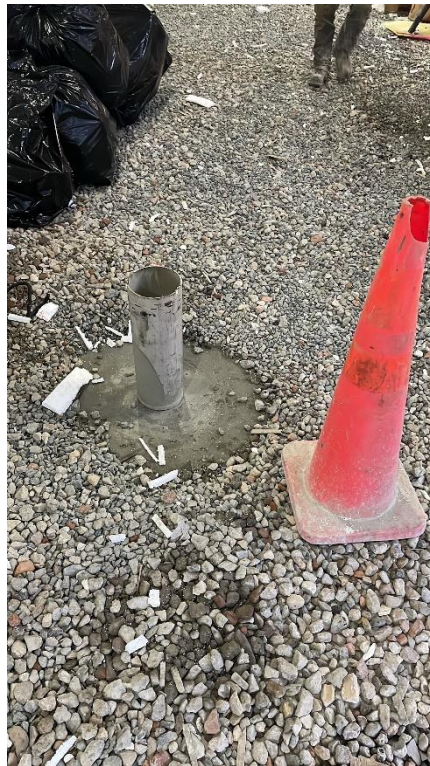
Photo 2: View of the casing set at MW-18D, facing south
