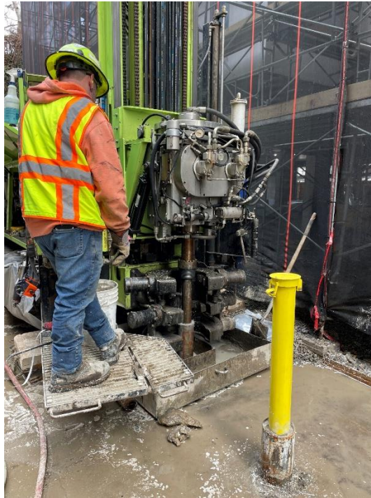
Photo 1: View of sonic drill rig setup on MW-9D, facing northeast
