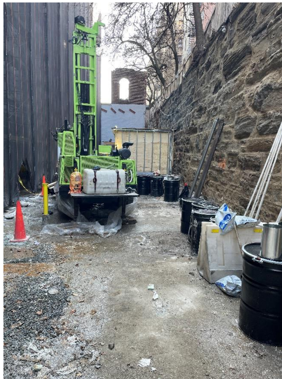
Photo 2: View of sonic drill rig setup on MW-16D to spin casing back down to completion depth, facing south
