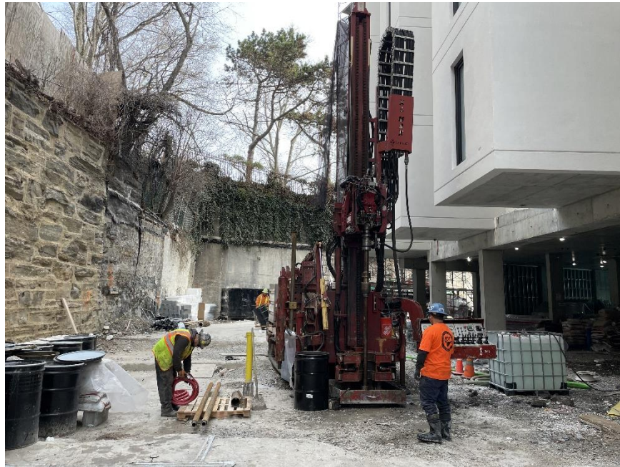
Photo 1: View of ADT advancing MW-09I, facing north.
