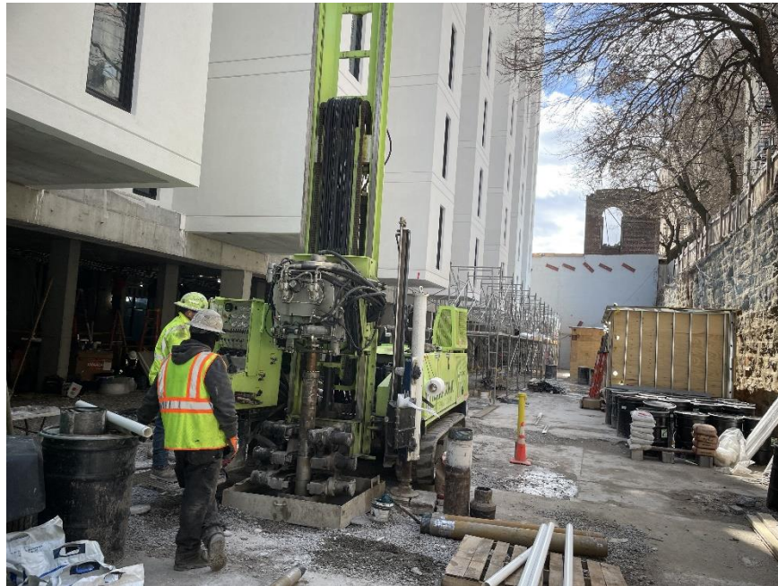
Photo 1: View of ADT advancing MW-14I, facing south.
