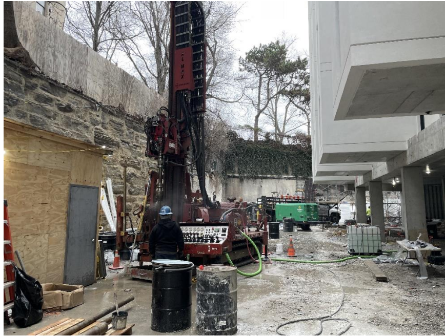
Photo 1: View of ADT advancing MW-16I, facing north.
