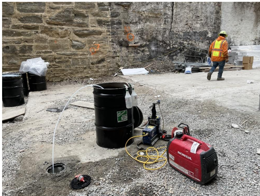
Photo 2: View of Haley & Aldrich developing MW-09S, facing west.
