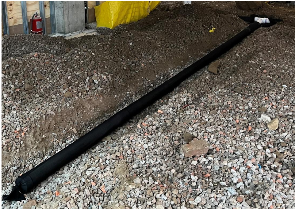
Photo 2: View of SSDS piping wrapped in non-woven geotextile fabric, facing southwest.
