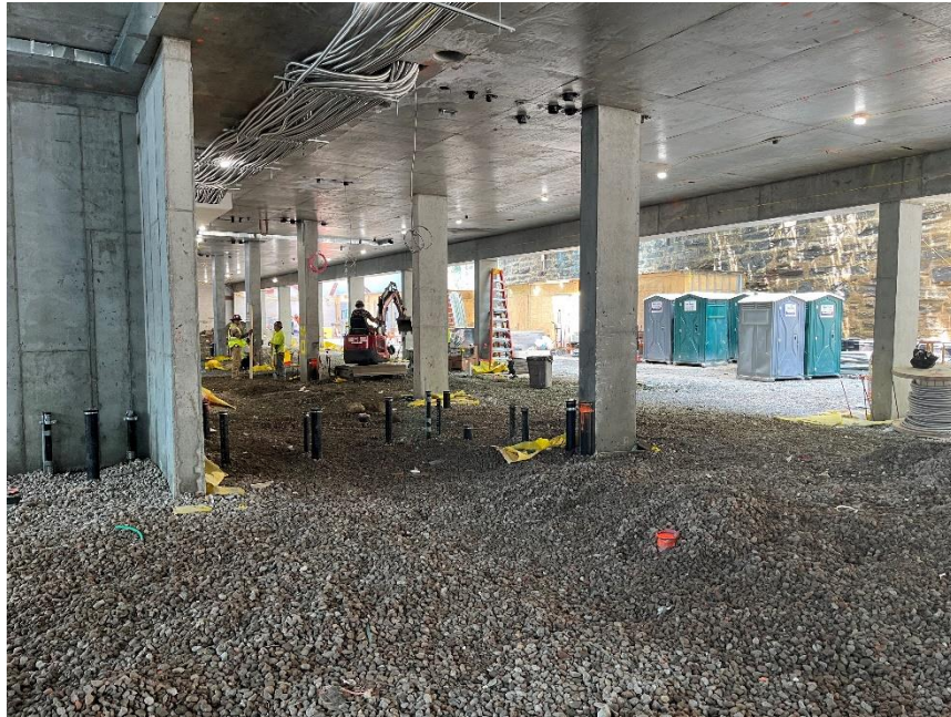
Photo 1: View of B Contractors burying the SSDS piping, facing southeast.
