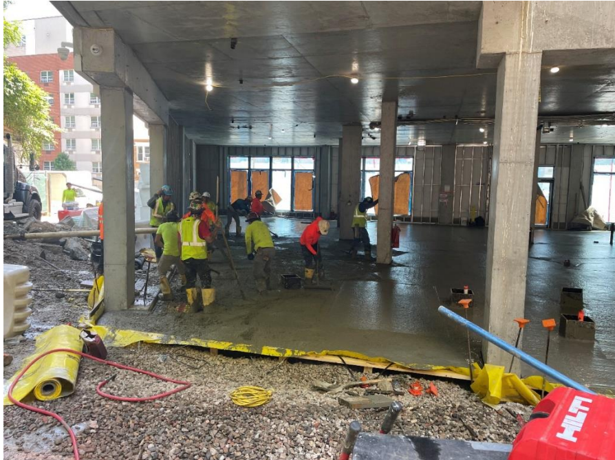
Photo 2: View of concrete pad installation, facing West.
