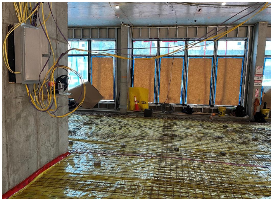
Photo 2: View of vapor barrier and metal mesh installation, facing east.
