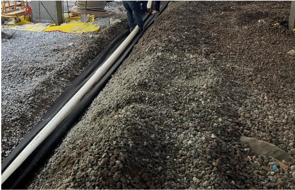
Photo 1: View of A & B Plumbing installing SSDS piping with geotextile fabric in the northwestern portion of the Site, facing north.
