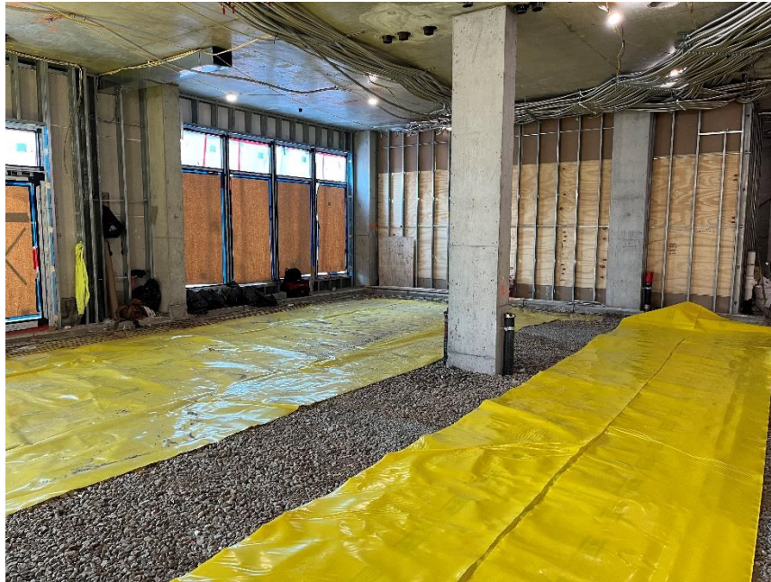
Photo 1: View of ongoing vapor barrier installation on the southeast portion of the site, facing southeast.
