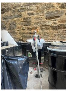
**Photo 1:** View of ISOTEC performing ISCO injection at MW-9S, facing west.
