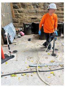
**Photo 1:** View of ISOTEC performing ISCO injection at MW-16D, facing west.
