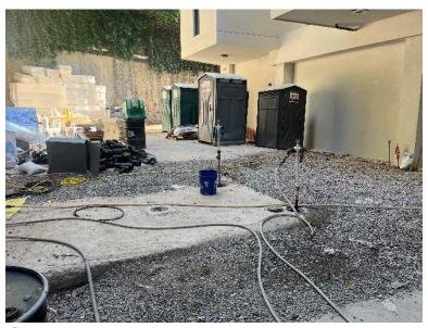
**Photo 1:** View of ISOTEC performing ISCO injection at MW-14S, facing north.
