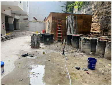
Photo 2: View of ISOTEC performing ISCO injection at MW-17I, facing south.
