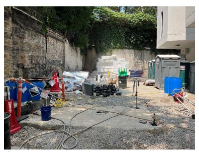
**Photo 1:** View of ISOTEC performing ISCO injection at MW-14I, facing north.
