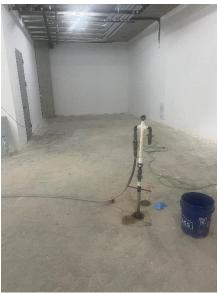
**Photo 2:** View of ISOTEC performing ISCO injection at MW-18S, facing south.
