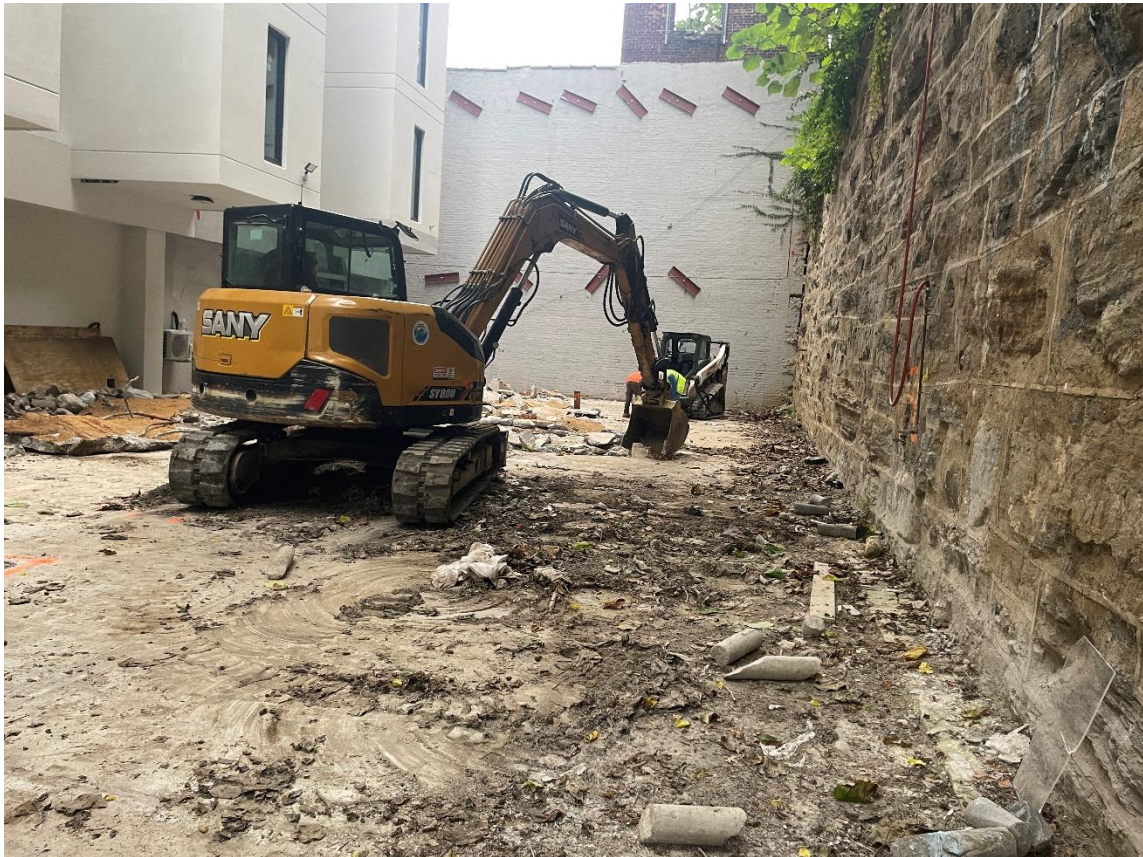
Photo 1: View of contractor breaking up existing driveway, facing south.
