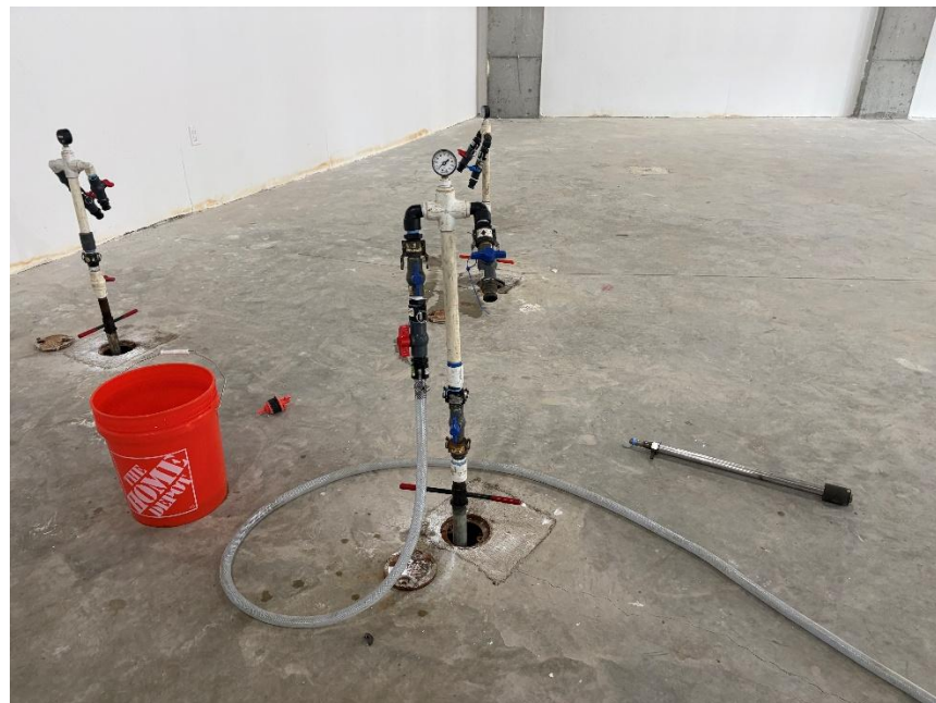
Photo 2: View of ISOTEC performing ISCO injection at MW-18S, facing north.
