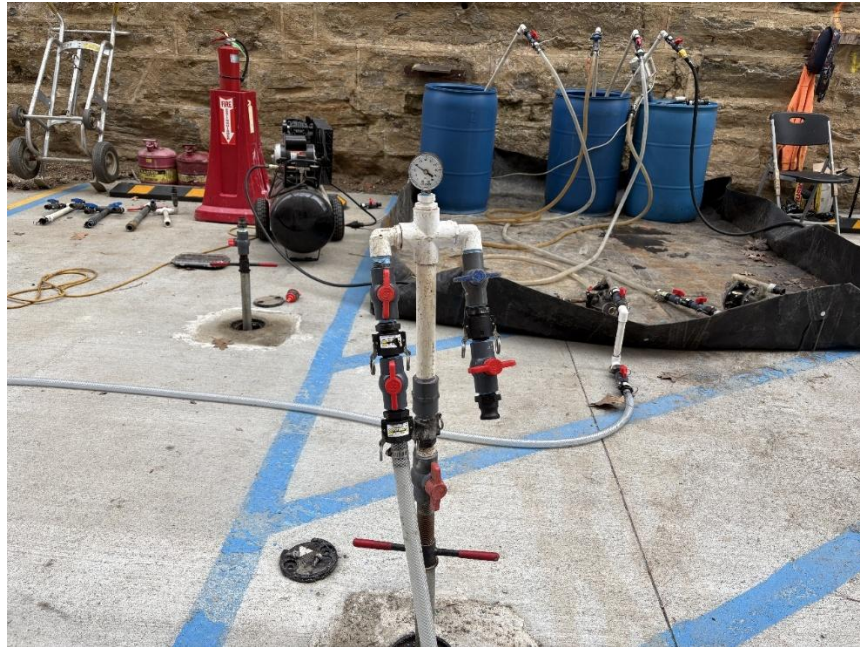
Photo 1: View of MW-16D injection site with ISOTEC's injection setup, facing west.
