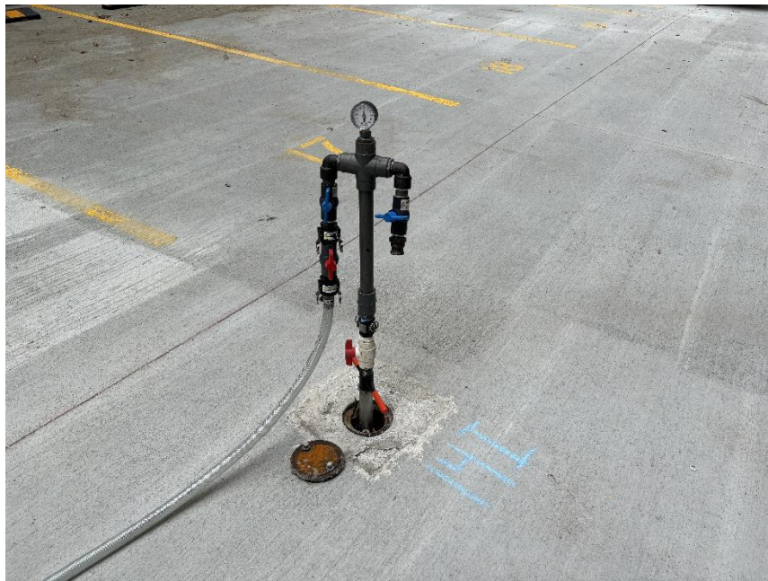
Photo 2: View of ISOTEC performing ISCO injection at MW-141, facing north.
