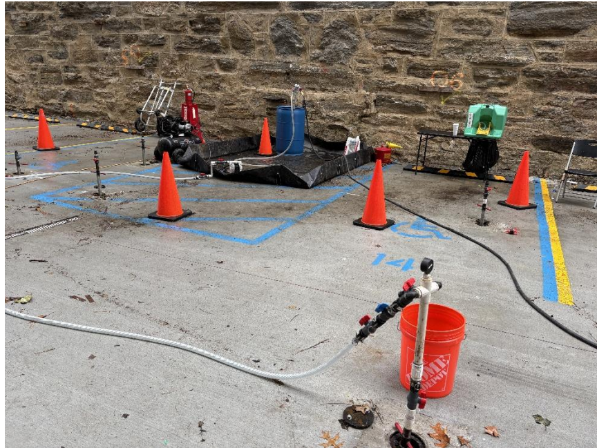
Photo 1: View of ISOTEC performing ISCO injection at MW-09I, facing southwest.
