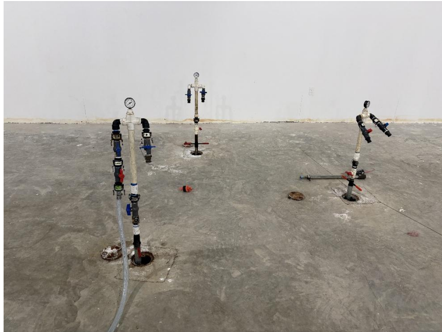
Photo 1: View of ISOTEC's performing ISCO injection at MW-18S, facing west.
