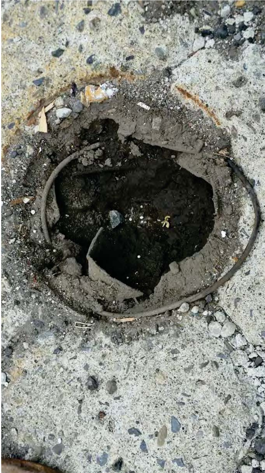
Photo 3: MW-10 well head. Casing/riser could not be found in manhole, even after exploratory digging.
