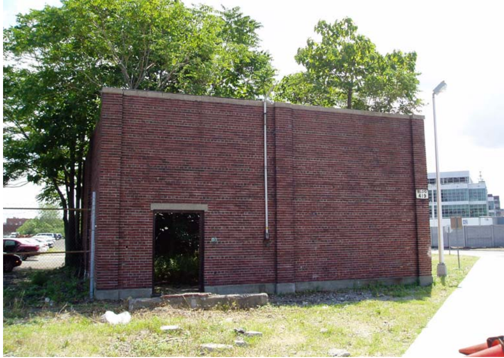
Exterior of Building #419
