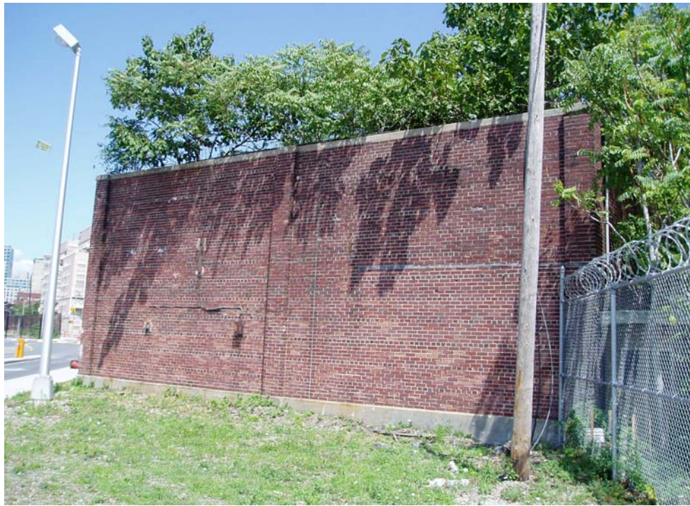
Exterior of Building #419
