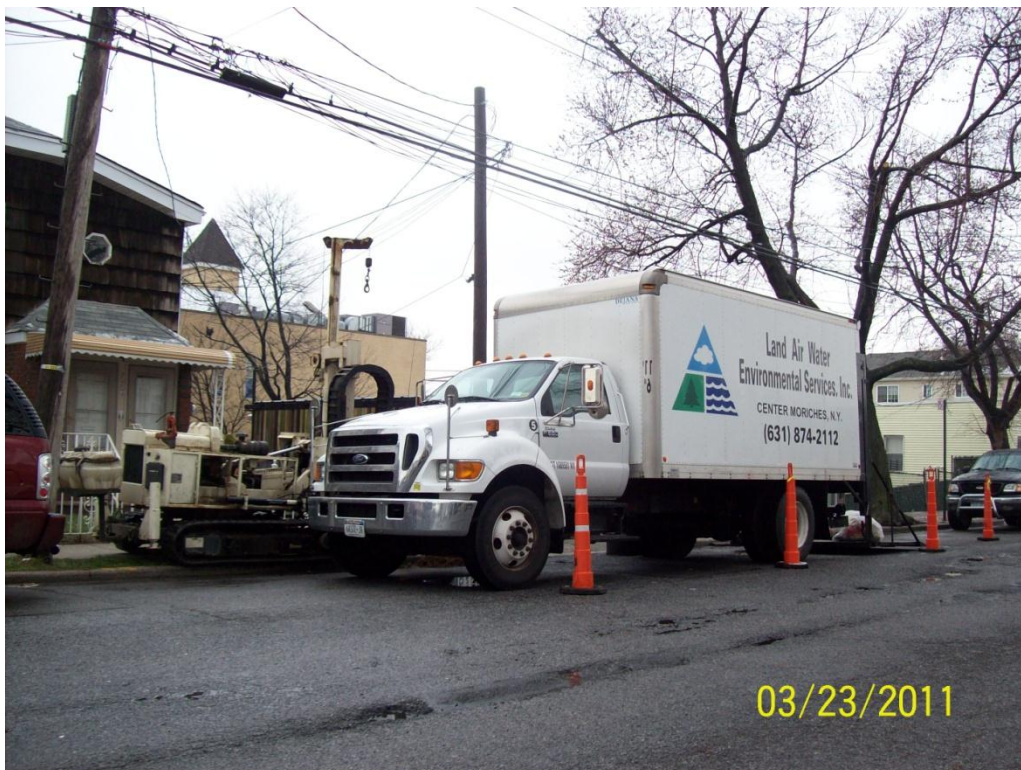
Photo 9. Installation of PZ-6 on the east side of Pine Street.
