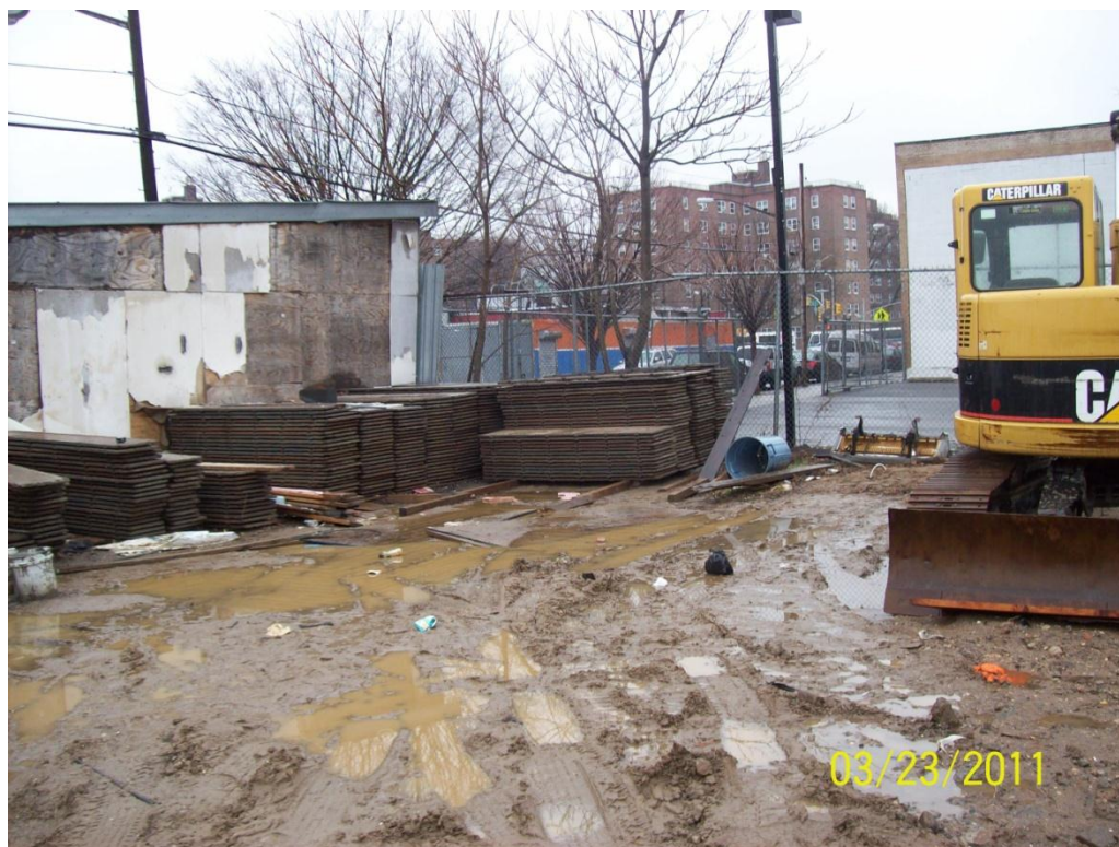
Photo 16. View of northwest corner of the site.
