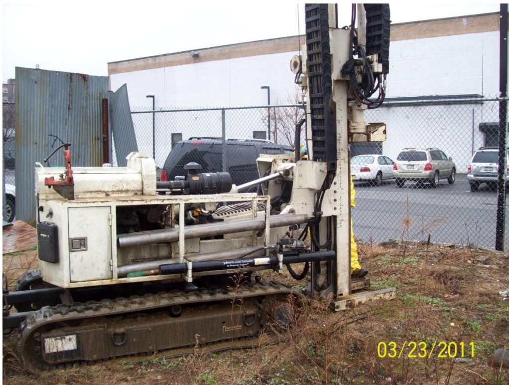
Photo 15. Installation of PZ-4R in the northern portion of the site.
