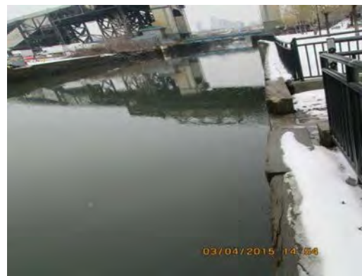
Looking North towards 9 th St. bridge bulkhead in front of Lowes
