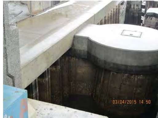
Facing Southeast at Lowes looking @ sheet piling bulkhead
