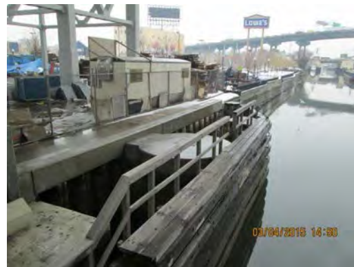
Looking South towards site looking at bulkhead
