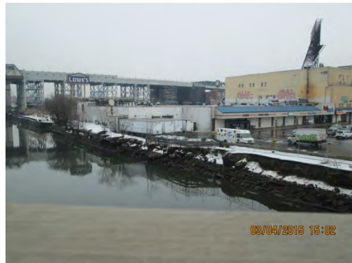
Looking Northeast towards site and Lowes and bulkhead
