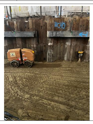
Photo 2: General backfill and compaction in WC-10 (C/D)
