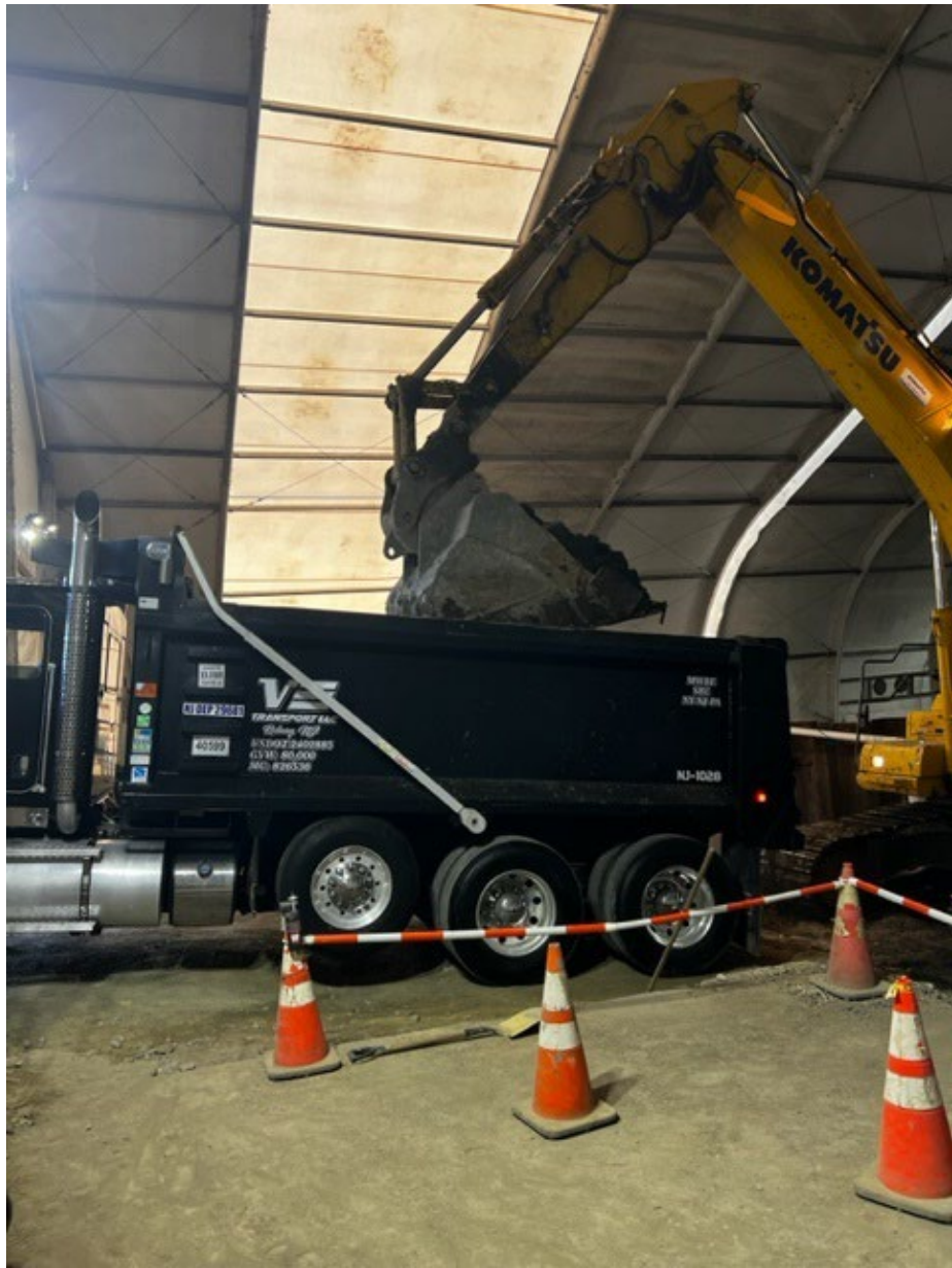
Photo 2: Load out of waste soils from WC-10
