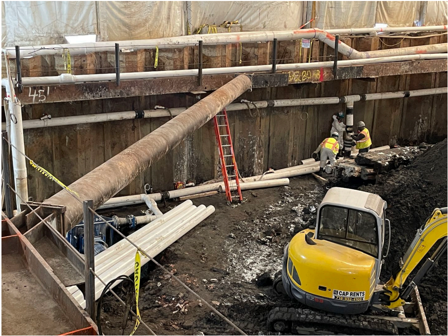
Photo 1: Looking northeast, view of ECS installing the new header pipe for well point recovery system in Gas Holder 3 excavation area.
