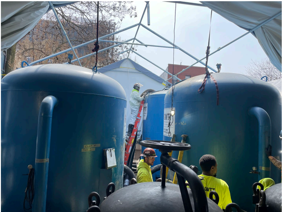
Photo 2: Looking south, view of CEI using a vacuum truck to remove spend carbon from train 2 of the water treatment system.
