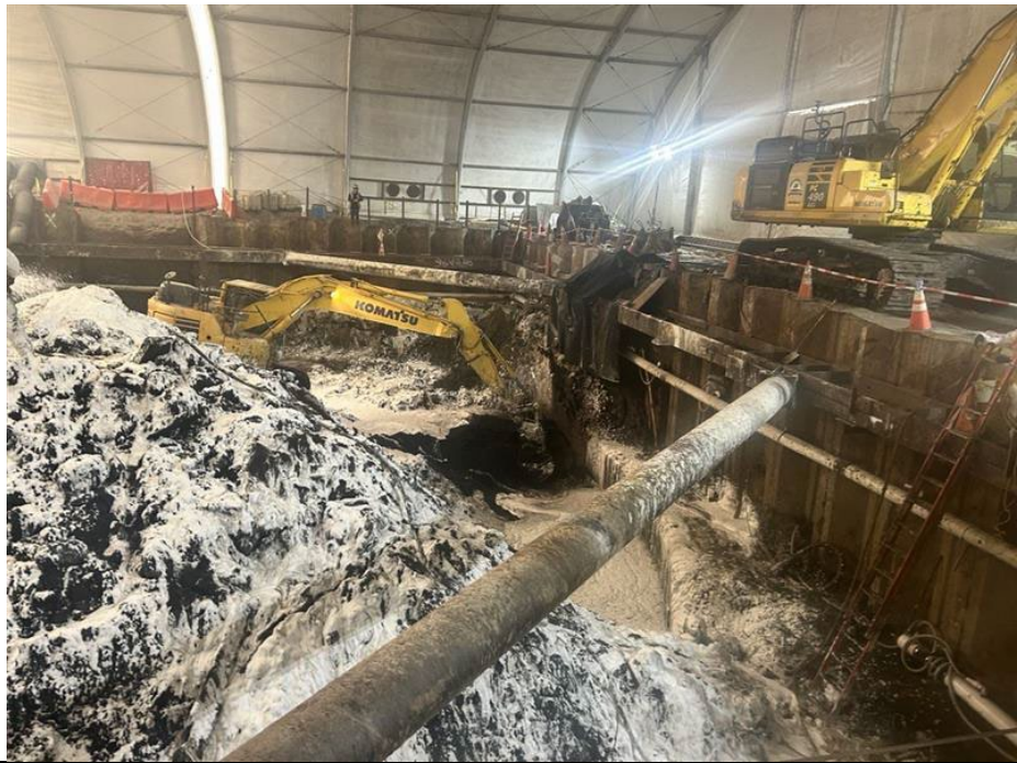
Photo 1: Looking east, view of CEI excavating in WC-GHE, demolishing former gas holder wall and stockpiling material for future load out.
