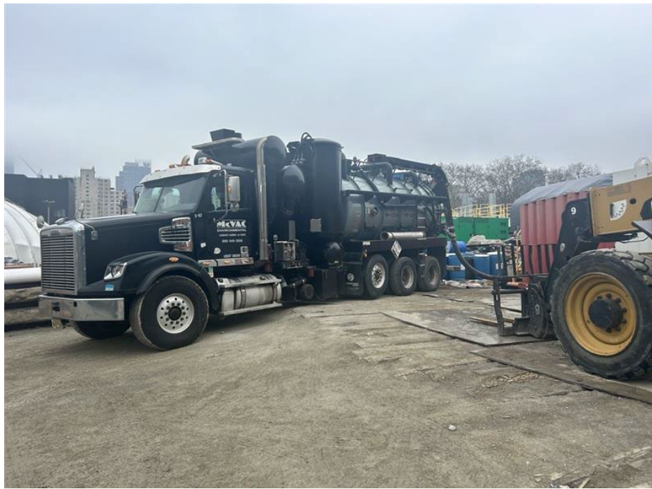
Photo 2: Looking south, view of CEI using vacuum truck to remove spent carbon from the lead carbon vessel of Train 2 of water treatment system.
