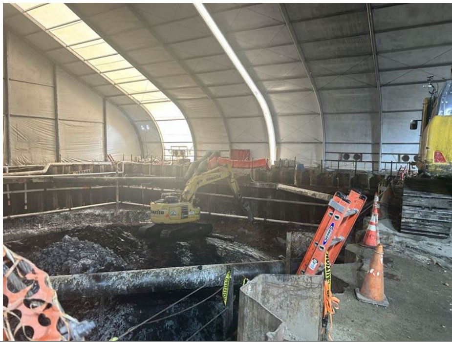
Photo 1: Looking northeast, CEI demolishes Gas Holder 3 walls in WC-GHE to elevation - 6.5' and prepares material for loadout and disposal.
