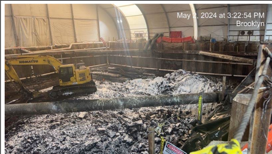
Photo 3: Looking northeast, CEI applying Atmos odor suppressant foam on exposed soil inside TFS to mitigate odors.
