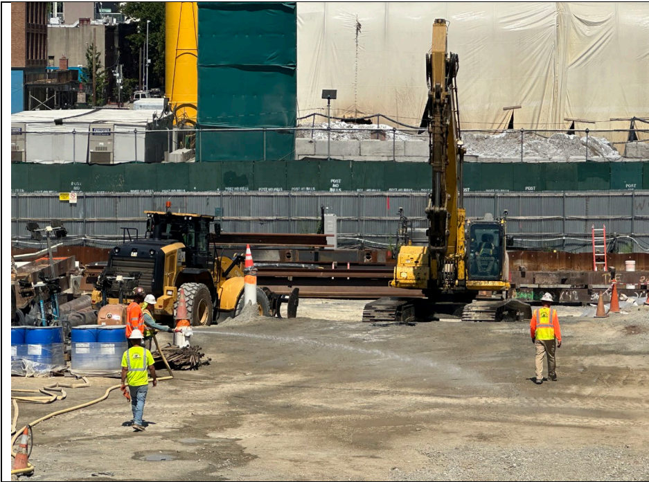
Photo 3: Looking west, view of CEI watering the work area to prevent dust.
