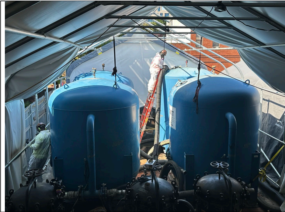
Photo 3: Looking south-southwest, view of CEI vacuuming spent filter media from the WTS via a vacuum truck.
