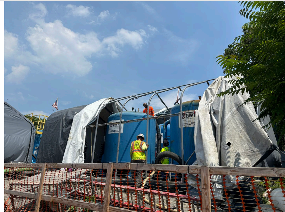
Photo 3: Looking east, view of CEI removing spent filter media from the WTS via a vacuum truck.
