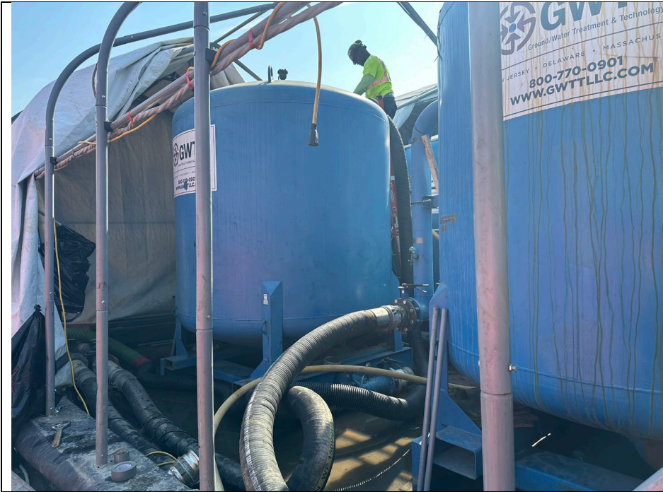
Photo 3: Looking northeast, view of CEI vacuuming spent filter media from the WTS via a vacuum truck.
