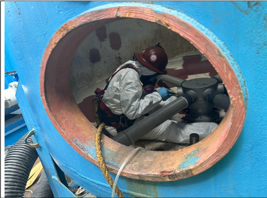
Photo 3: Looking west, view of GWTT replacing previously damaged screens from a WTS vessel.
