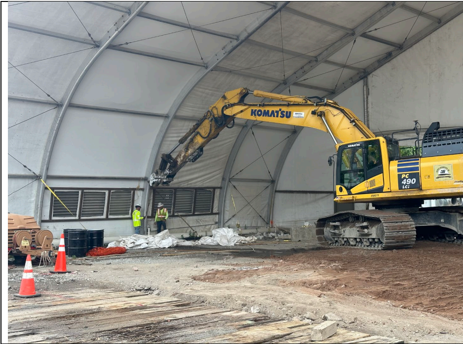
Photo 3: Looking southwest, view of CEI removing steel pins from the base plates in preparation of relocation of the TFS.
