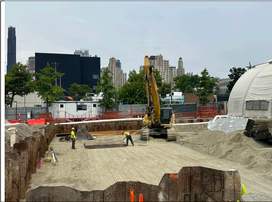
Photo 3: Looking north, view of CEI leveling material and placing crane mats within former Gas Holder 3 area to facilitate crawler crane installation for upcoming sheet pile removal activities.
