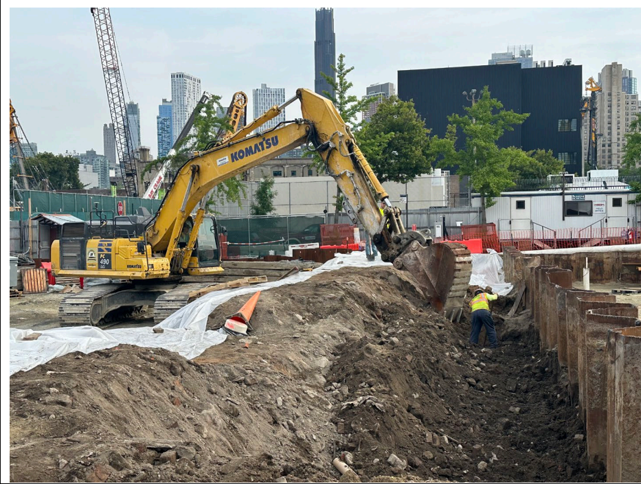
Photo 1: Looking north, view of CEI sloping soil benched against steel sheet piles along the western perimeter of former Gas Holder 3 excavation area.
