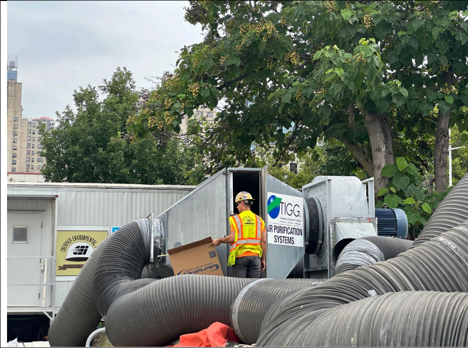
Photo 2: Looking northeast, view of CEI changing the filters from the VMS blowers.
