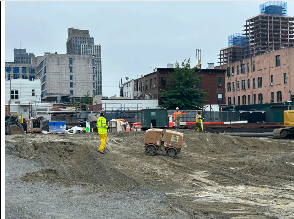
Photo 3: Looking southwest, view of CEI compacting backfill material previously imported from Vulcan Wantage Quarry southwest of former Gas Holder 3 excavation area.
