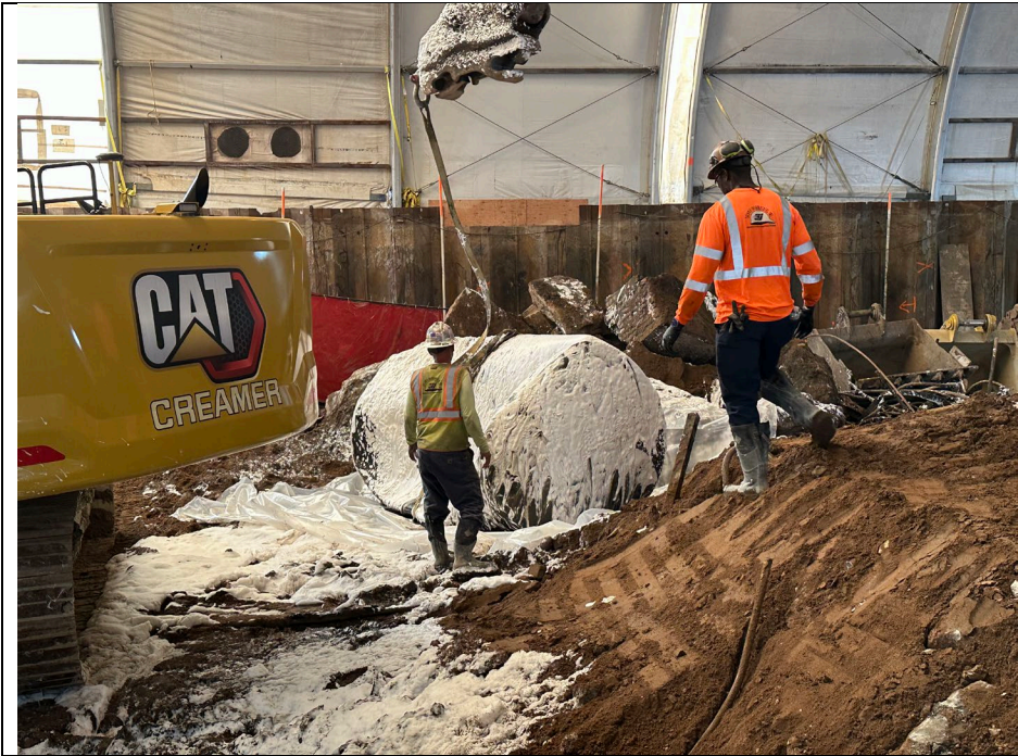
Photo 3: Looking east, view of CEI temporarily relocating the discovered UST within waste characterization grid WC-GH4-1.
