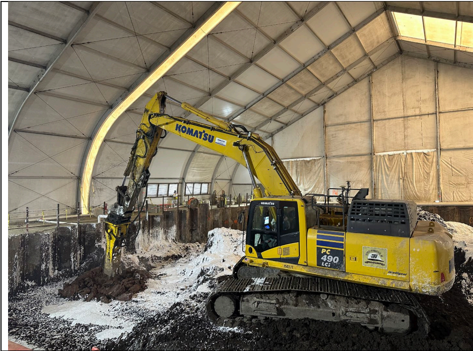
Photo 3: Looking north, view of CEI breaking the former Gas Holder 4 wall within the southwest corner of the excavation area.
