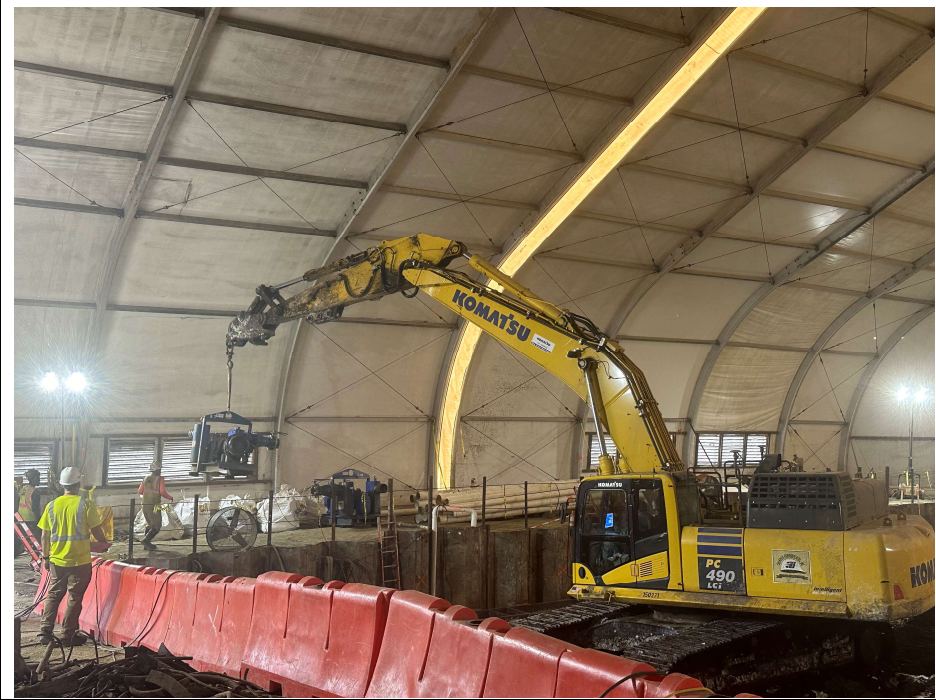
Photo 3: Looking northwest, view of CEI assisting ADG with mobilization of vacuum pumps for the upcoming wellpoint header pipe installations.
