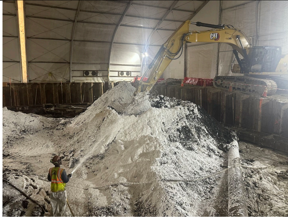
Photo 3: Looking southeast, view of CEI applying Atmos odor suppressing foam within the Gas Holder 4 excavation area during loadout activities.
