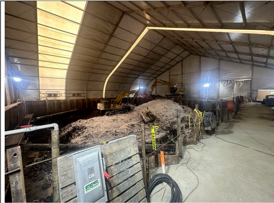
Photo 3: Looking southeast, view of CEI applying Atmos odor suppressing foam within the Gas Holder 4 excavation area during soil handling activities.
