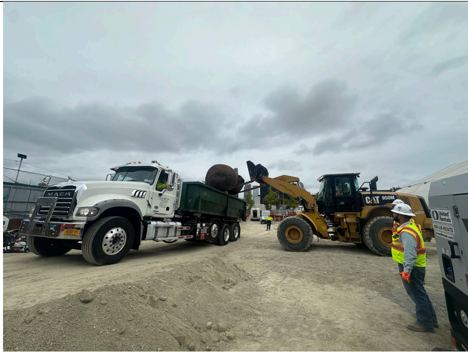
Photo 3: Looking north, view of ENTACT and AARCO loading the previously cleaned UST for offsite disposal.
