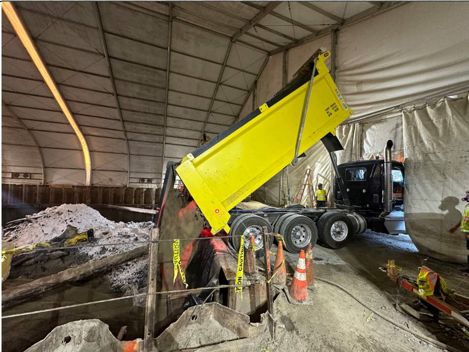
Photo 2: Looking southeast, view of a triaxle truck unloading general fill material within the Gas Holder 4 excavation area.
