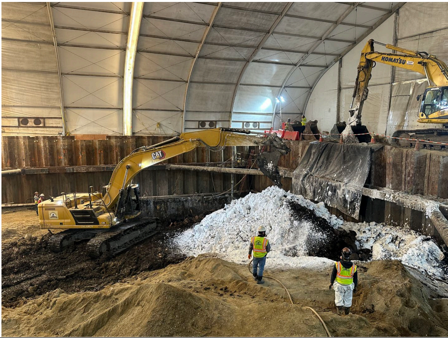
Photo 3: Looking east-southeast, view of CEI applying Atmos odor suppressing foam during excavation activities.
